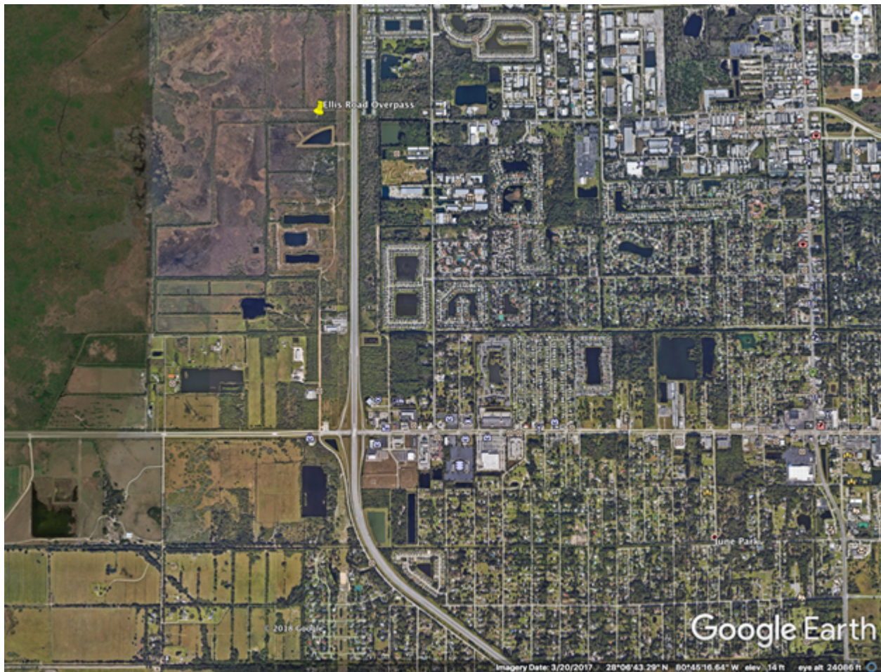
Figure 3-16 Google Earth Pro Image of Ellis Road Overpass
