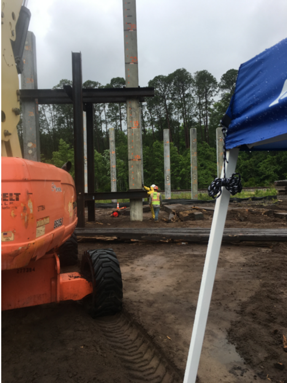
Figure 3-7 Photo of Baldwin Bypass North Bound End Bent 4 Pile 1
