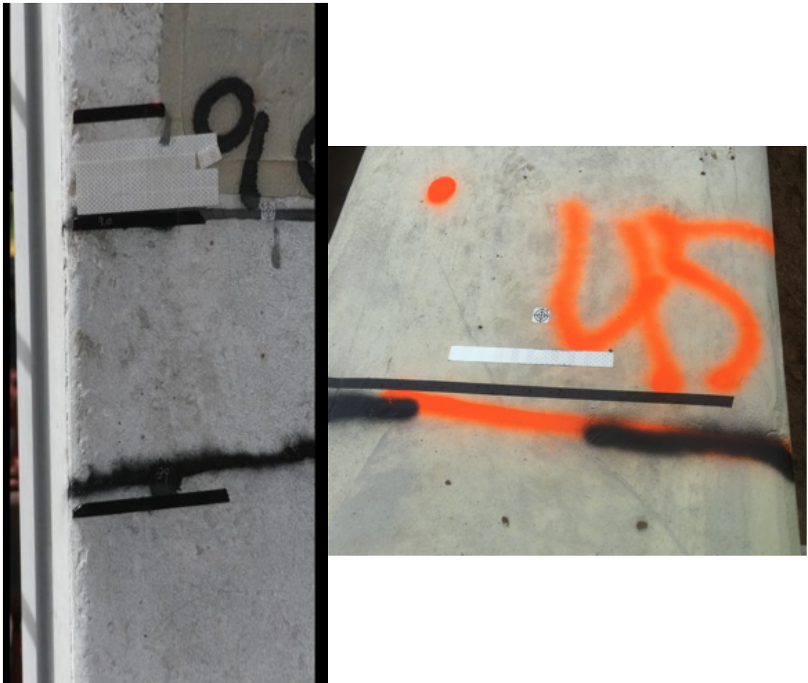
Figure D-3 Typical Pile plus PDM Markings
