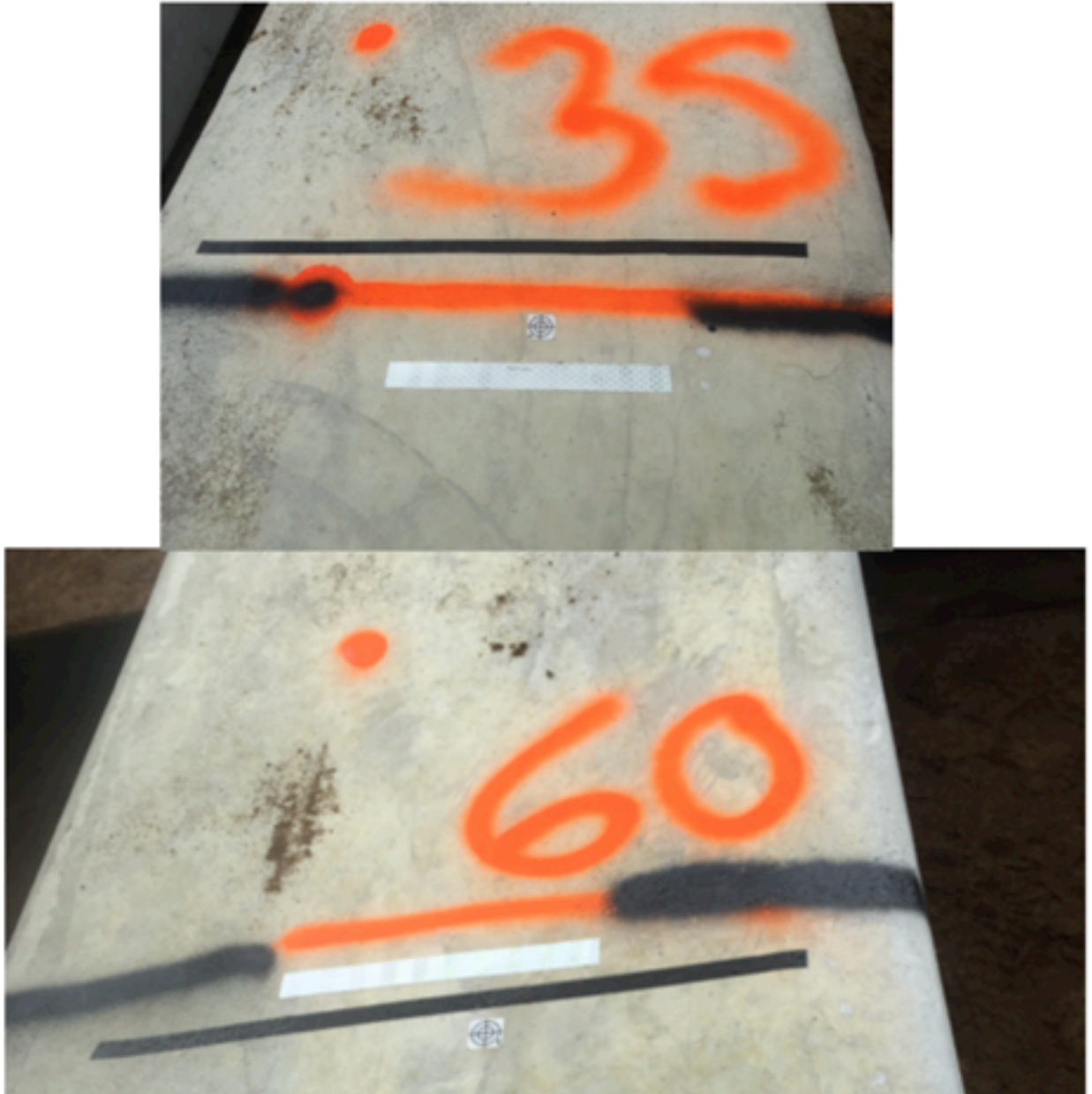
Figure 6-4 Baldwin Bypass PDM and CMS 5-foot spacing pile markings
