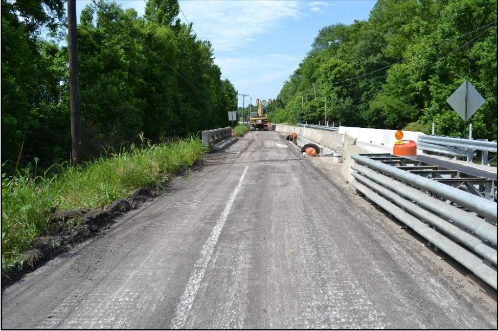
Figure 4-1: Bridge No. 94-SR11-0.87
