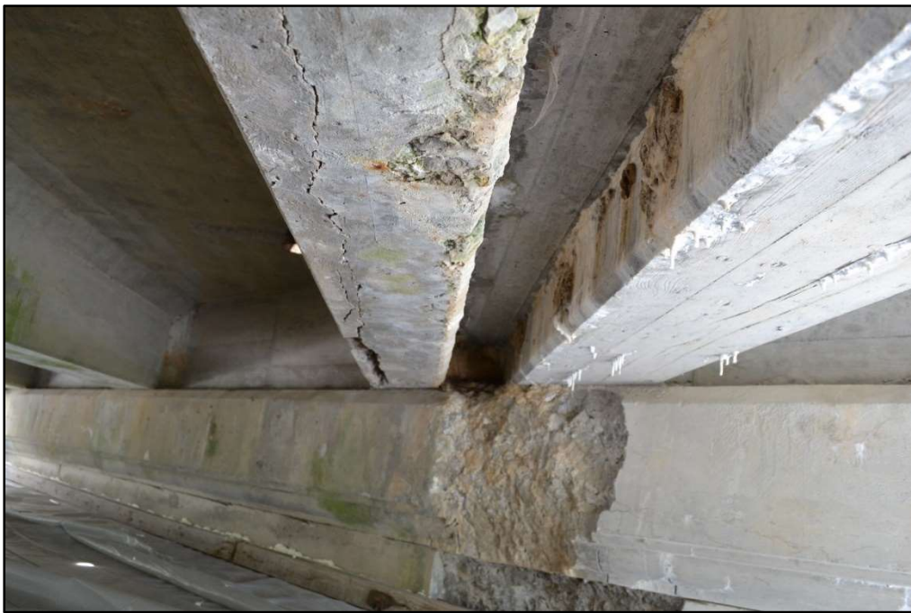
Figure 4-18: Superstructure - Deterioration
