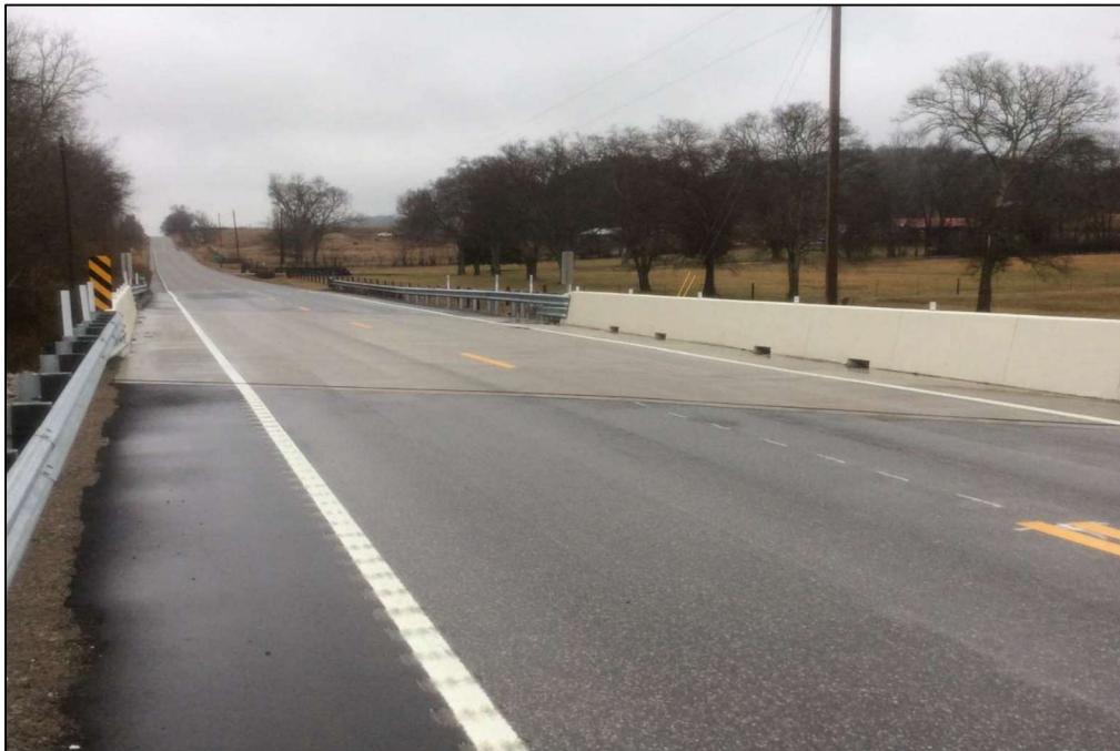
Figure 4-48: Completed Deck – Bridge No. 94-SR11-0.59
