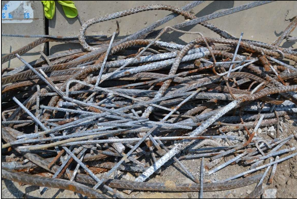
Figure 4-3: Reinforcing Removed During Demolition
