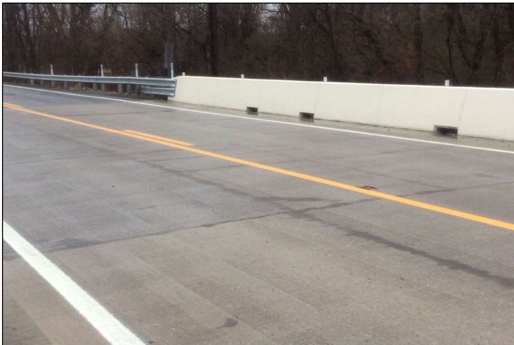
Figure 4-58: Completed Deck – Bridge No. 94-SR11-0.87
