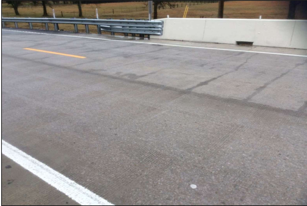
Figure 4-53: Completed Deck – Bridge No. 94-SR11-0.59
