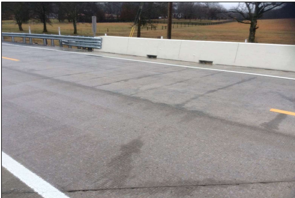
Figure 4-52: Completed Deck – Bridge No. 94-SR11-0.59
