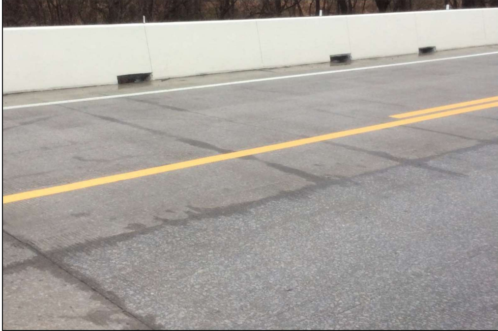
Figure 4-63: Completed Deck – Bridge No. 94-SR11-0.87
