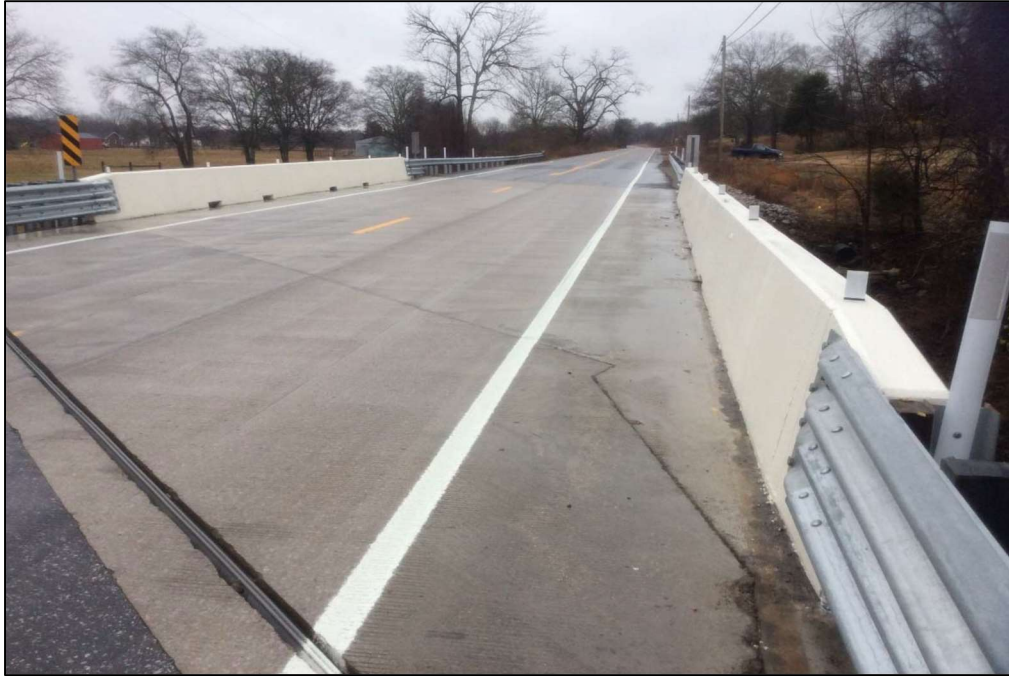
Figure 4-55: Completed Deck – Bridge No. 94-SR11-0.59
