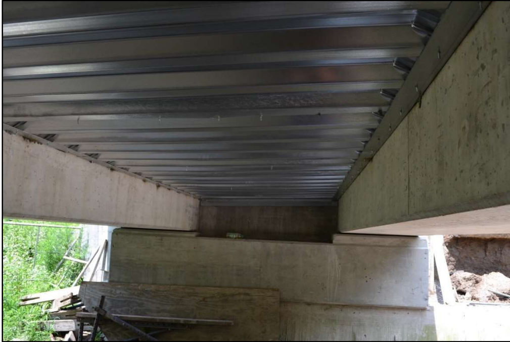
Figure 4-37: Deck – Form Installation
