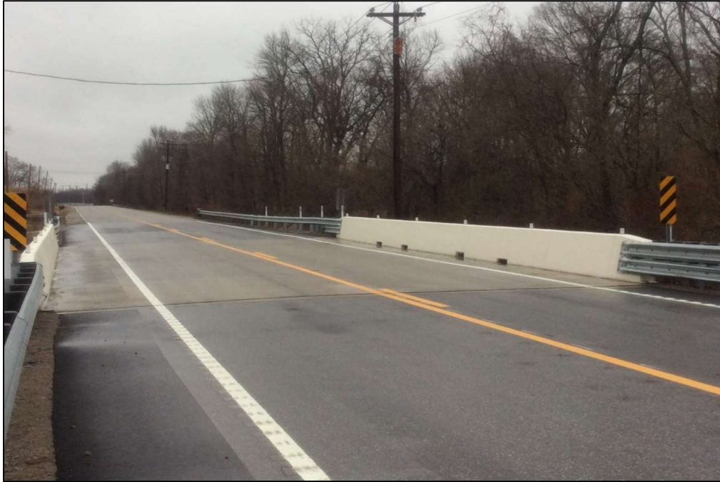
Figure 4-57: Completed Deck – Bridge No. 94-SR11-0.87
