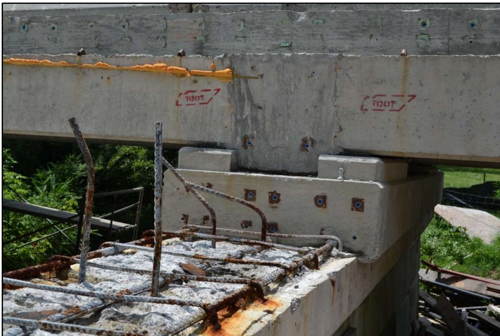
Figure 4-26: Superstructure – Completed Phase
