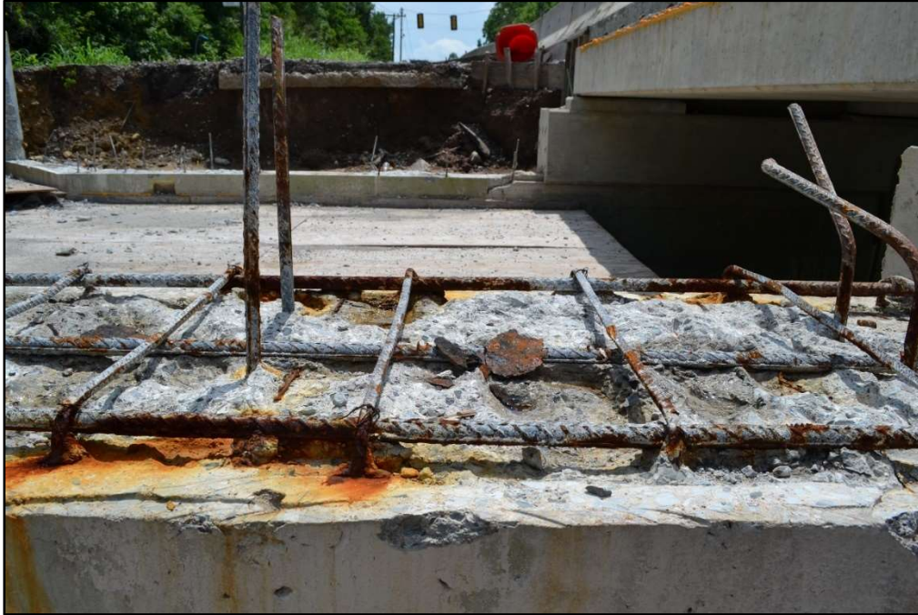
Figure 4-13: Substructure – Prepared for Modification
