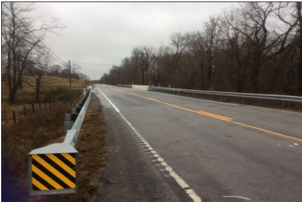
Figure 4-56: Completed Deck – Bridge No. 94-SR11-0.87
