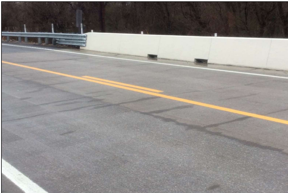
Figure 4-60: Completed Deck – Bridge No. 94-SR11-0.87
