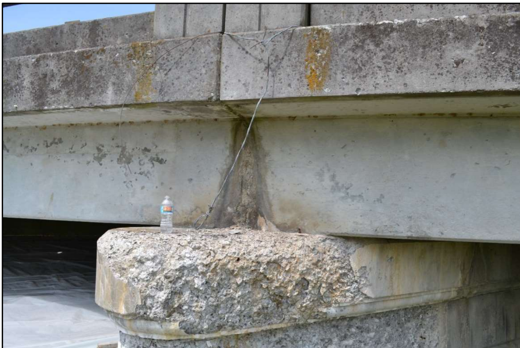
Figure 4-6: Substructure – Deterioration
