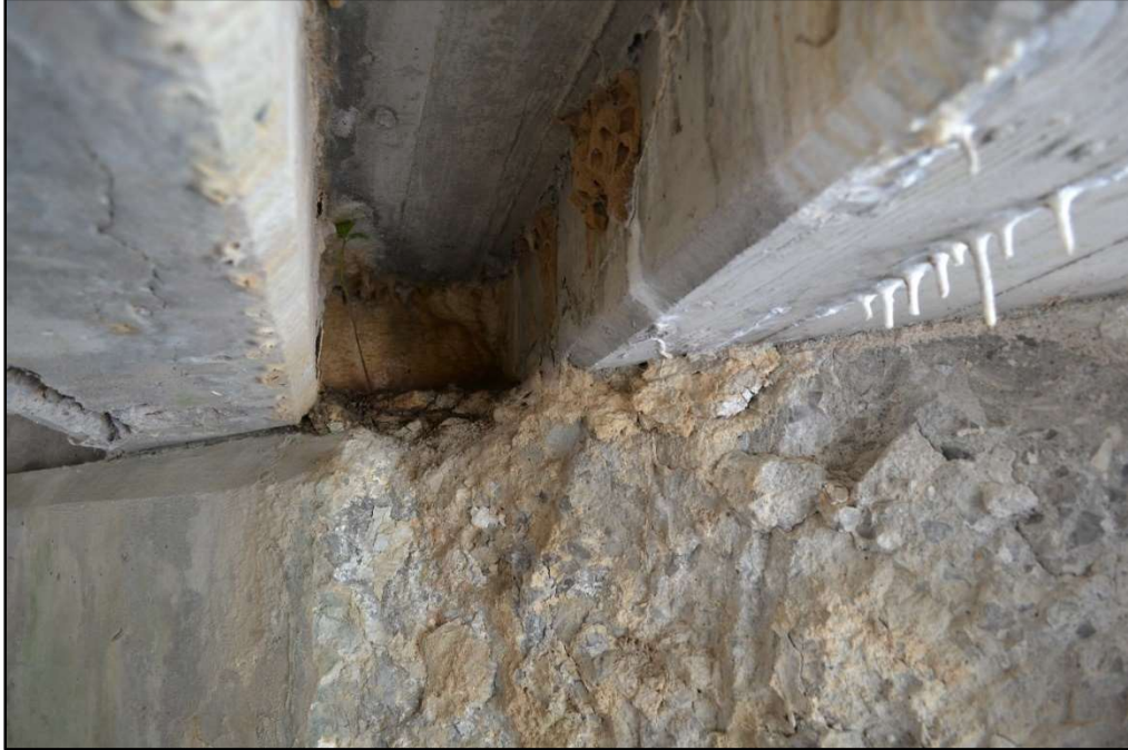
Figure 4-5: Substructure – Deterioration
