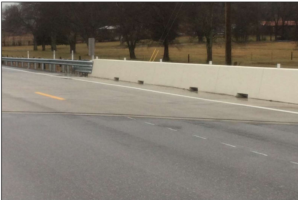
Figure 4-46: Completed Deck – Bridge No. 94-SR11-0.59
