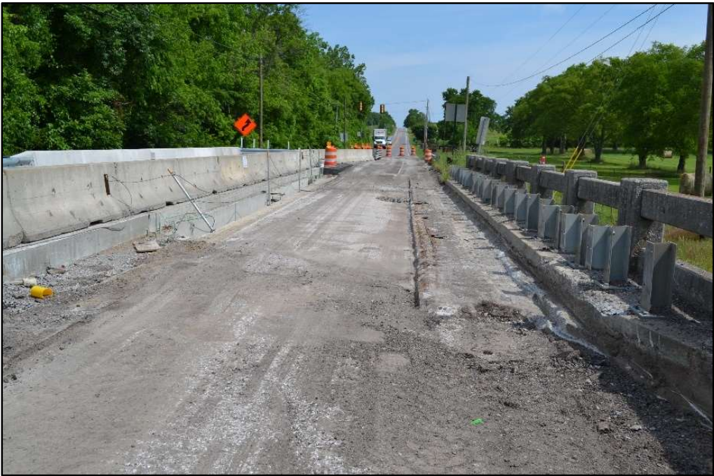
Figure 4-2: Bridge No. 94-SR11-0.59
