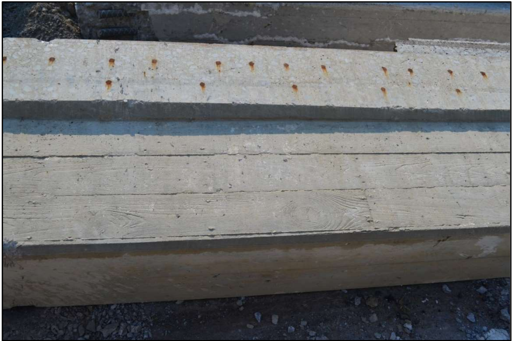
Figure 4-34: Deck – Cross Section After Removal
