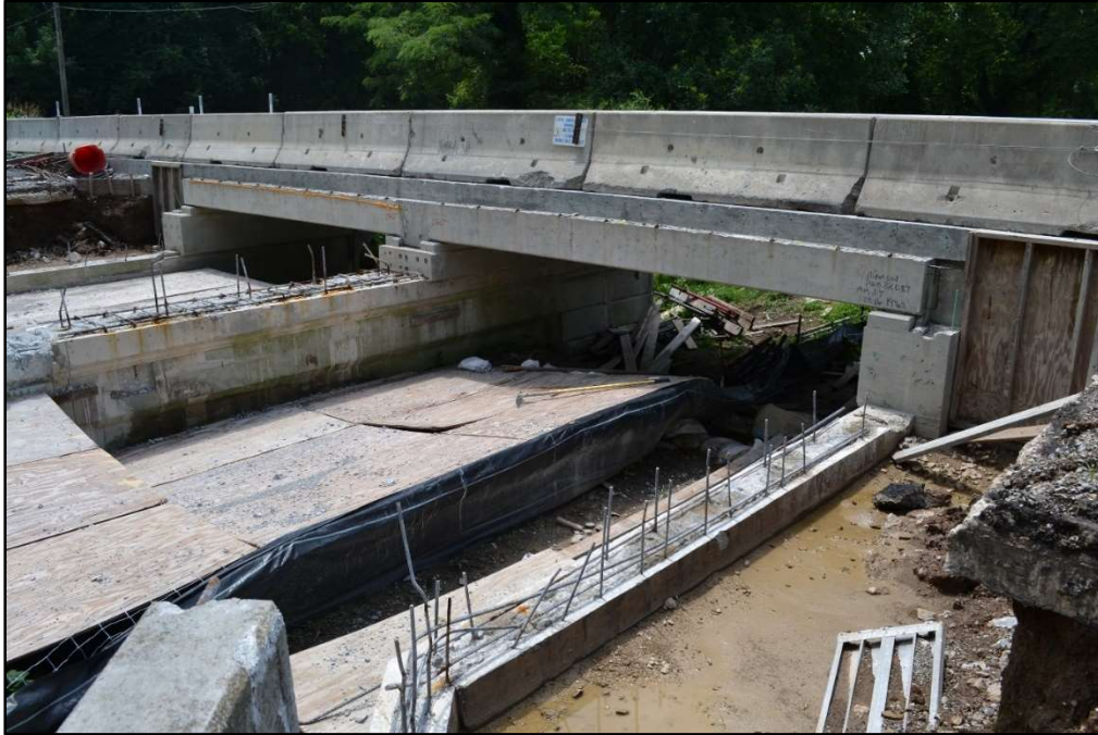
Figure 4-25: Superstructure – Completed Phase
