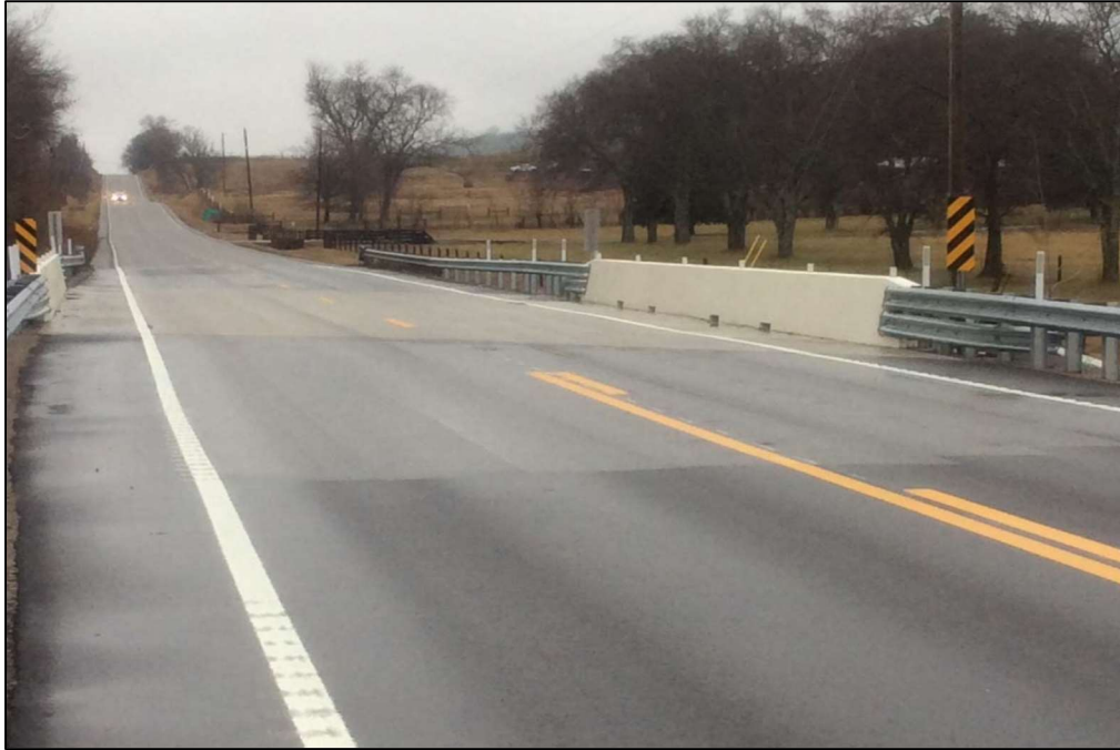
Figure 4-45: Completed Deck – Bridge No. 94-SR11-0.59
