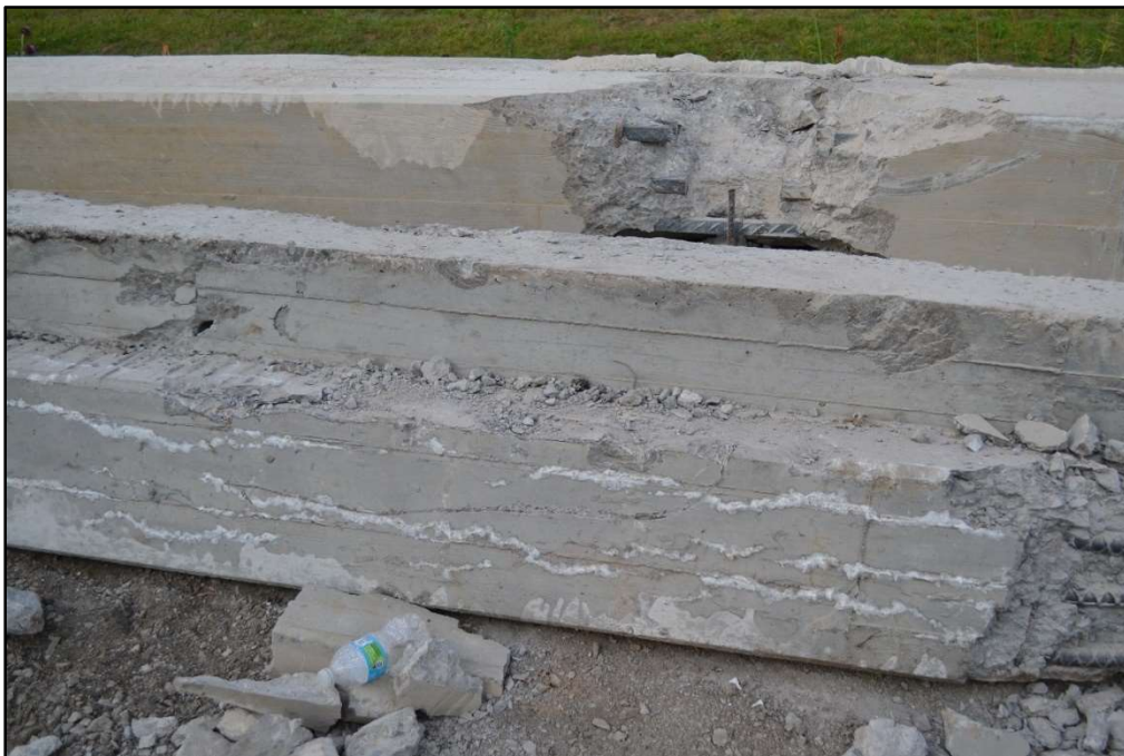
Figure 4-22: Superstructure - Deterioration
