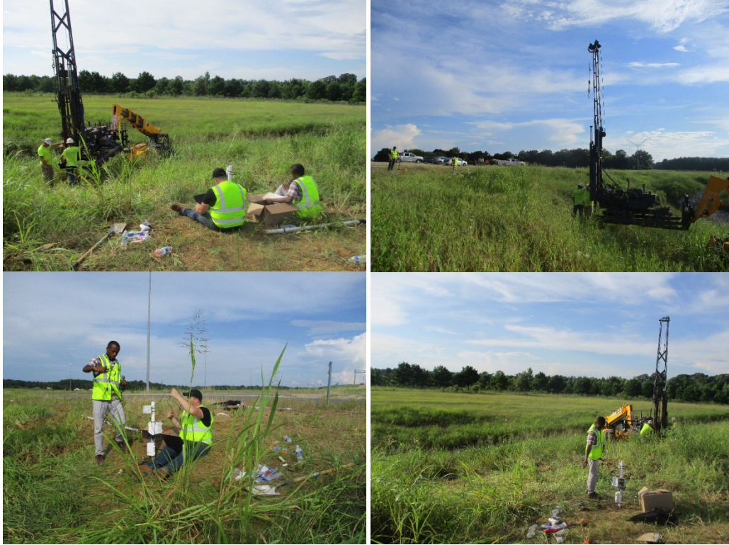
Figure 4.48 Installation of sensors at Slope 5
