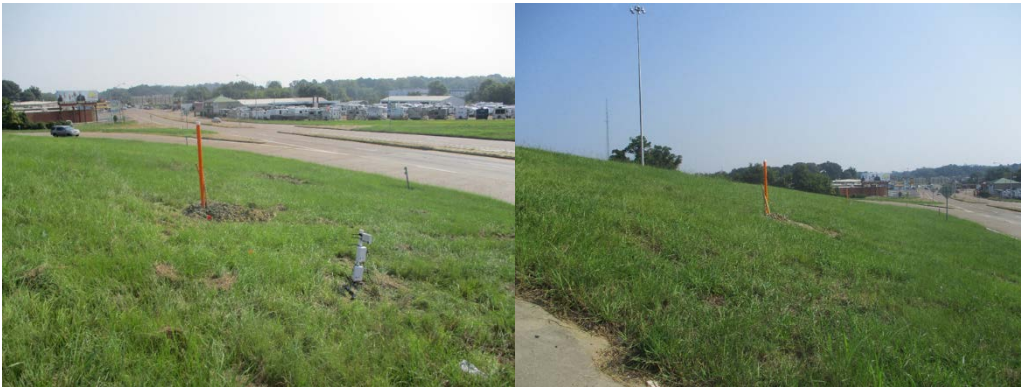
Figure 4.28 Inclinometer casting at Slope 3
