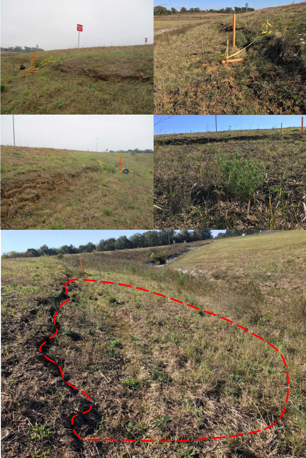
Figure 4.53 Landslides at Slope 5
