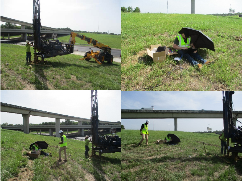
Figure 4.5 Slope 1 sensor installation
