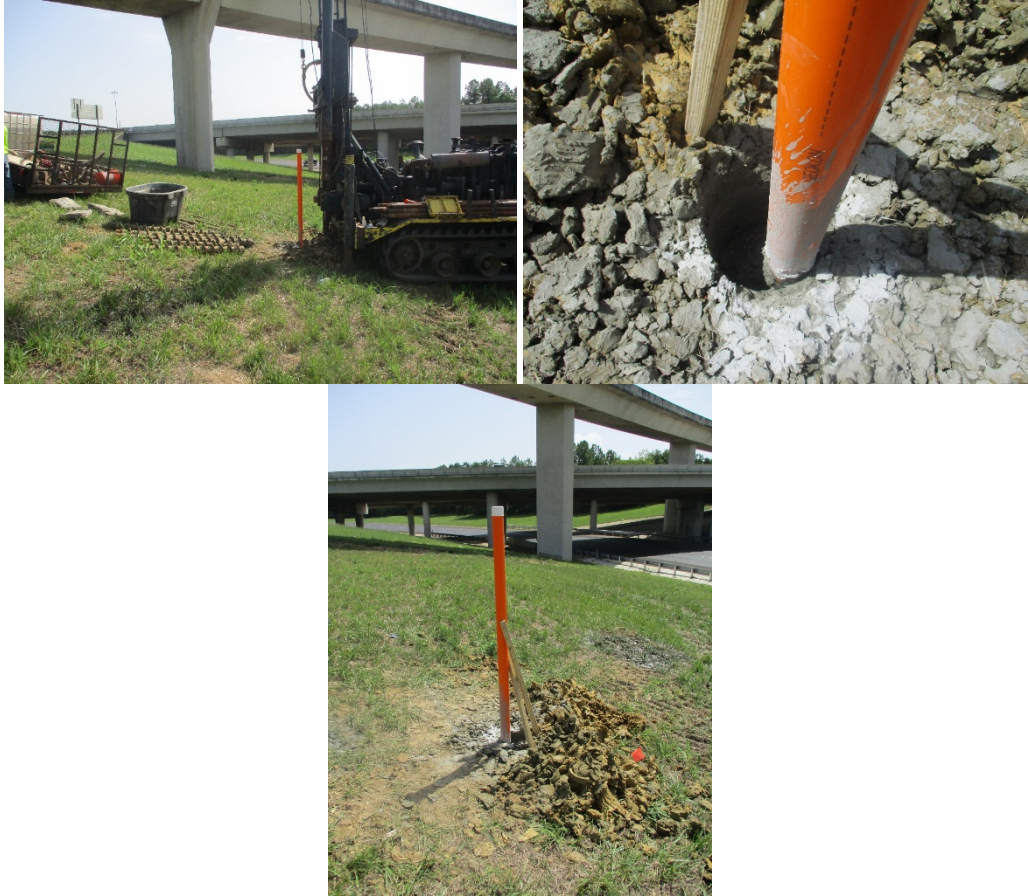
Figure 4.6 Slope 1 slope inclinometer installation
