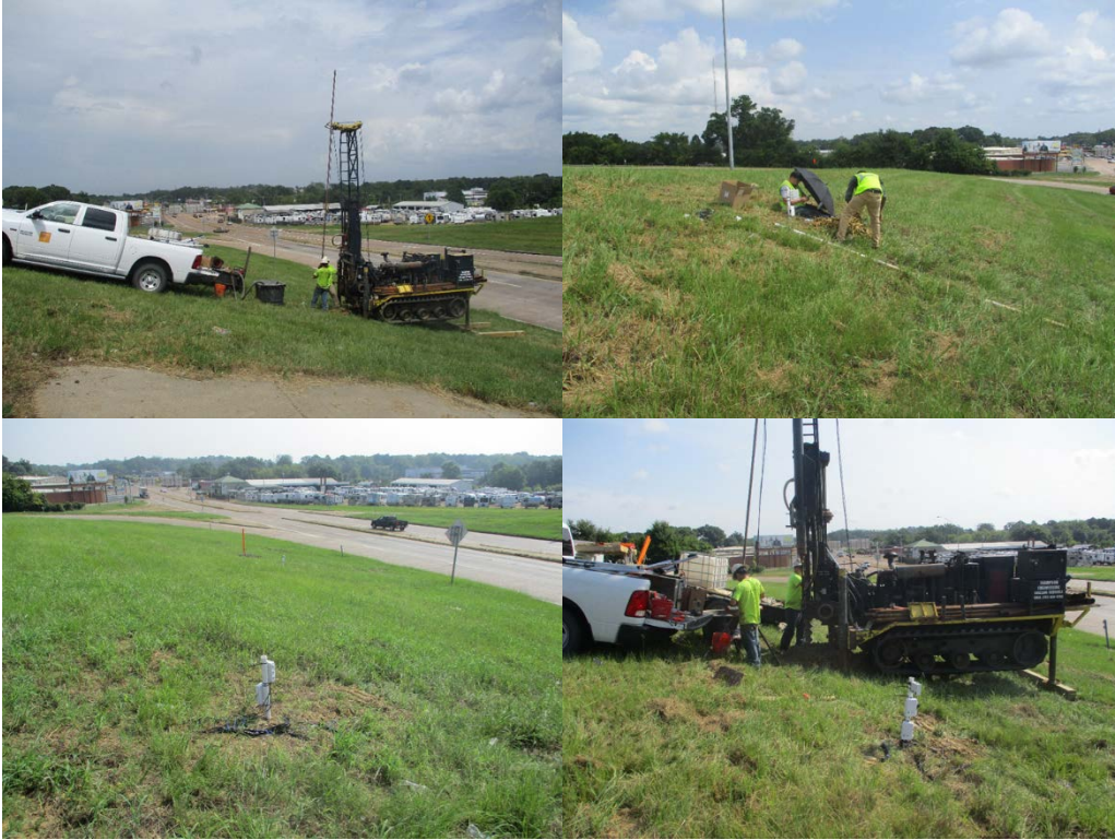
Figure 4.27 Field Instrumentation Activities at Slope 3
