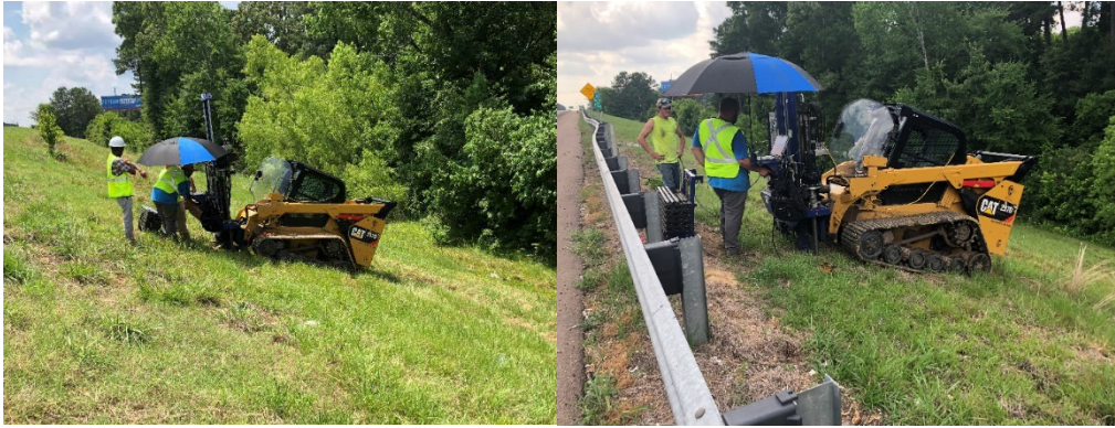
Figure 3.26 Field activity of CPT at Slope 4
