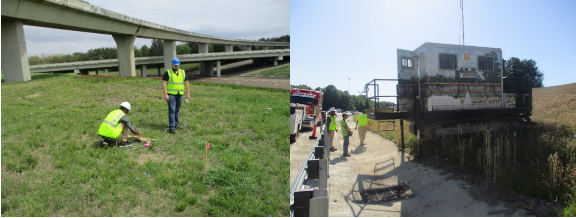
Figure 3.3 Conducting CPT test at Slope 1
