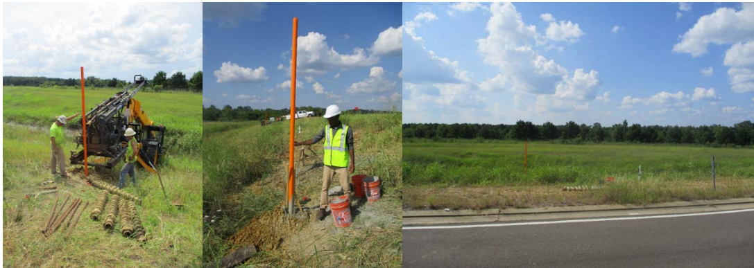
Figure 4.49 Slope 5 slope inclinometer installation
