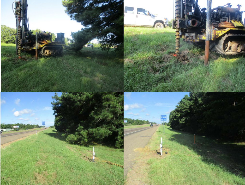
Figure 4.59 Slope 6 sensor installation
