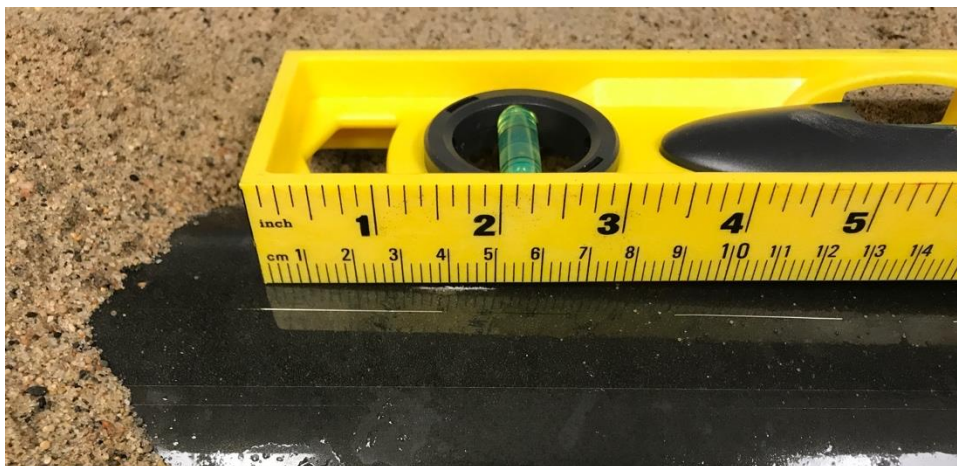
Figure 88. Distance measurement between crack and Sensor 2/Sensor 3.
