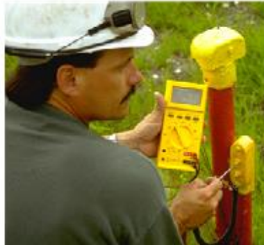
Figure 44. Field measurement example for pipe-to-soil potential 15 .
