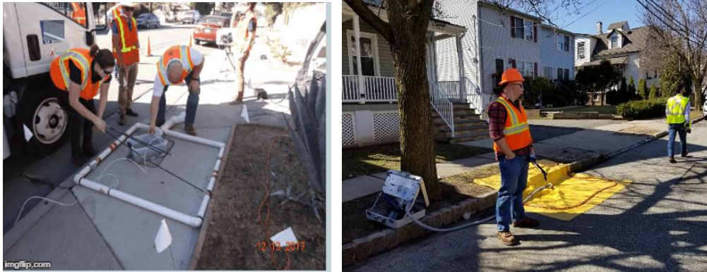
Figure 5 – Immediately following the technology providers methane emission quantification, surface expression quantification is performed
