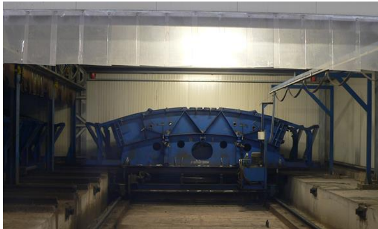
Figure 5-3: Segment mold at the Galleria Sparvo. Photo: FHWA.
