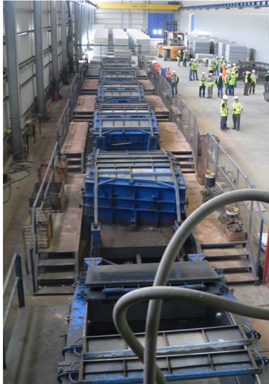
Figure 5-2: Segment mold carousel at the concrete plant of the Galleria Sparvo. Photo: FHWA.
