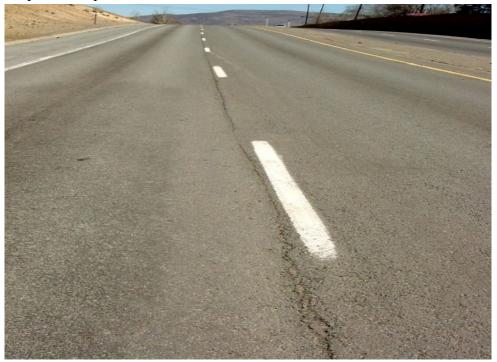
Image: Adam Hand Figure 1. Deteriorating Longitudinal Joint.
