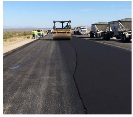
Image: University of Nevada Reno Figure 12. Bridging by Pinching with Drum on Cold Mat on the First Roller Pass.
