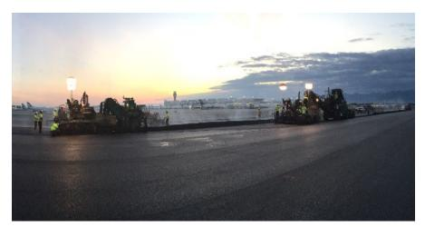
Image: Adam Hand Figure 7. Echelon Paving Operation.
