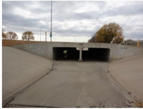
Twin Barrel Box Culvert
