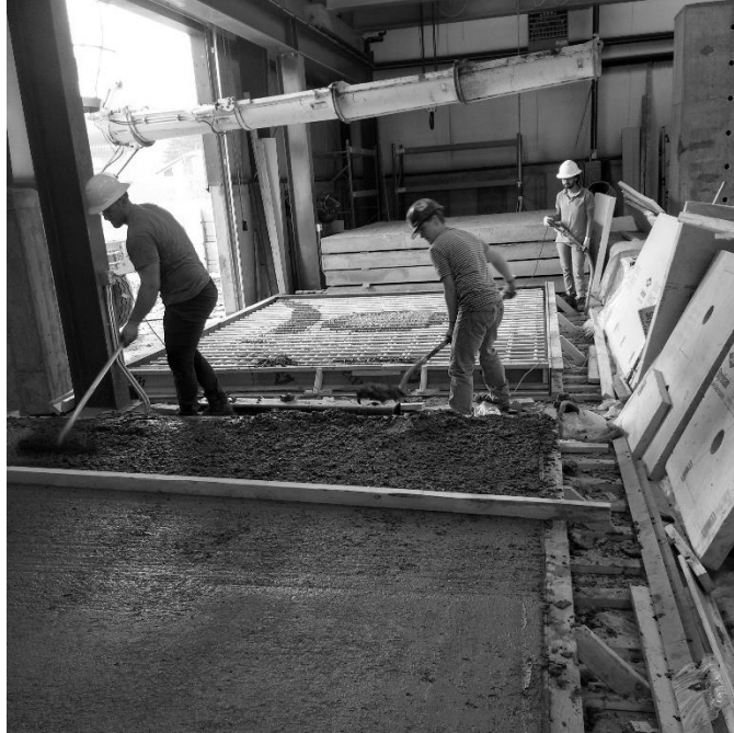
Figure 4.3.5 Pouring the GFRP punching shear decks
