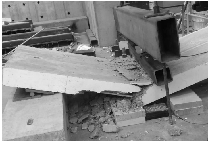
Figure 7.4.13 Side view of 1 million cycle GFRP specimen at failure
