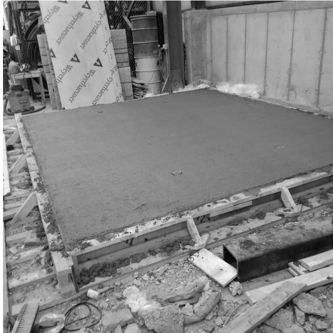
Figure 4.3.8 Finished GFRP punching shear deck
