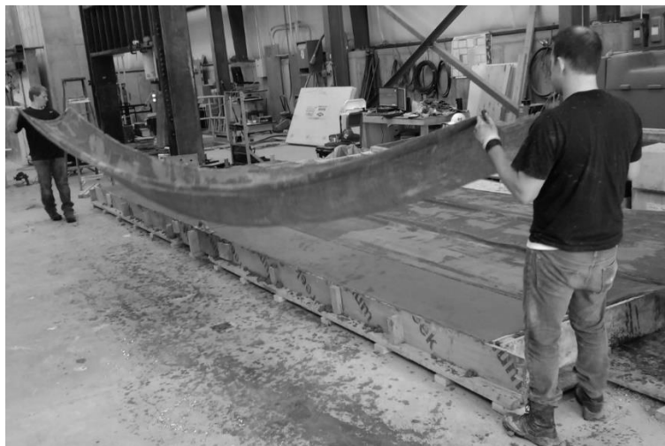
Figure 3.3.7 Laying moist burlap on the panels
