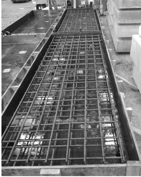
Figure 3.3.6 Steel-reinforced decks prior to pouring
