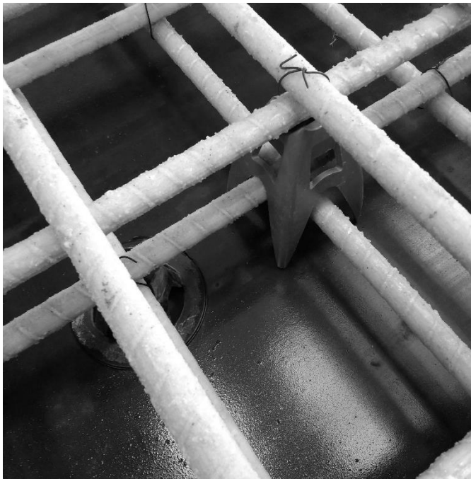
Figure 4.3.4 Close-up of GFRP reinforcement on chairs prior to pouring
