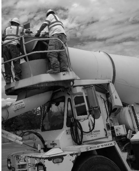
Figure 4.3.1 Adding the fibers at the batch plant
