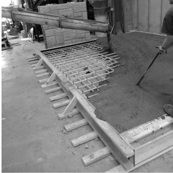
Figure 4.3.7 HRC decks being poured with internal vibration
