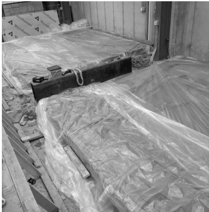
Figure 4.3.9 Curing the punching shear decks
