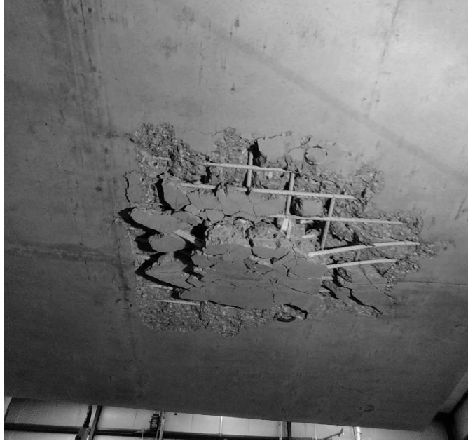
Figure 8.2.10 Bottom surface of GFRP punching shear deck
