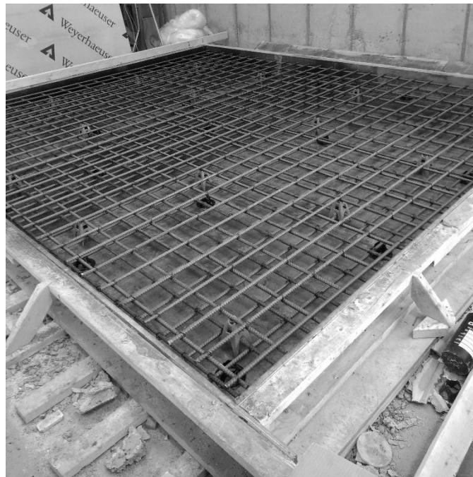
Figure 4.3.2 Steel punching shear deck prior to pouring
