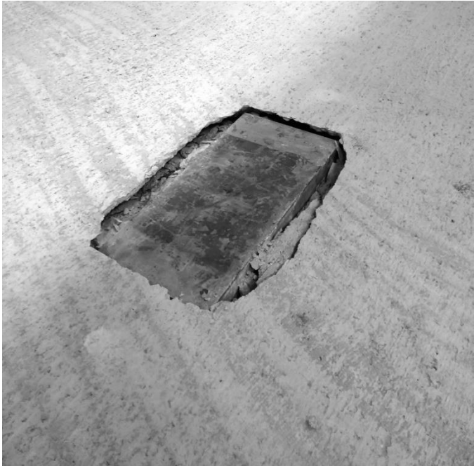
Figure 8.4.5 Top of steel post-fatigue punching shear deck
