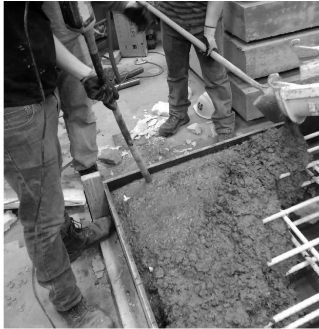
Figure 3.3.5 Internal vibration of deck panels
