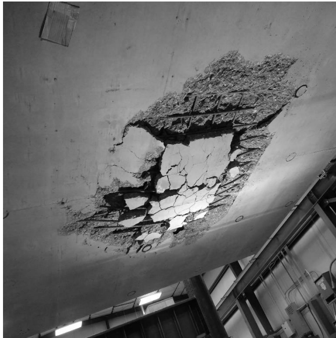
Figure 8.2.9 Bottom surface of steel punching shear deck
