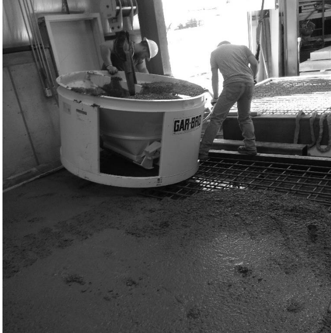
Figure 4.3.3 Pouring the steel punching shear deck with concrete hopper
