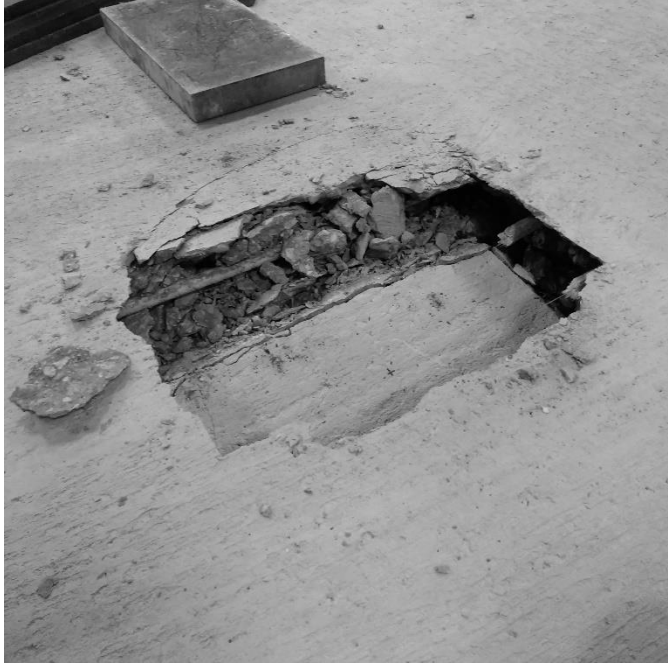
Figure 8.2.6 Top of GFRP punching shear deck
