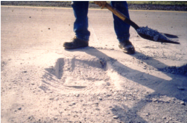
Figure 7b. Milled patch with rounded edges.
