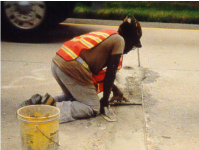
Figure 26. Finishing the patch.
