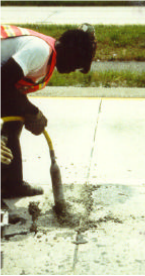
Figure 24. Using an internal vibrator.
