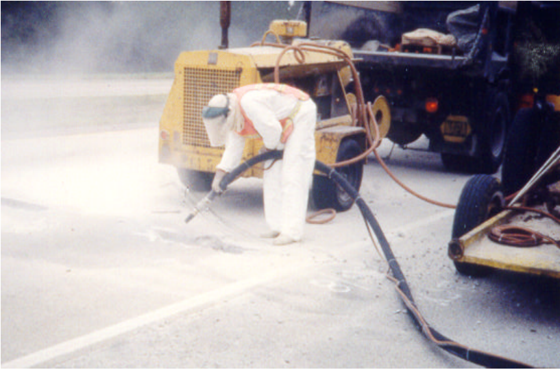
Figure 17. Sandblasting.
