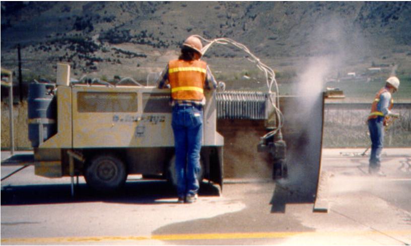
Figure 16. Protective shield around waterblasting operation.
