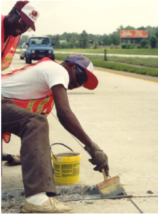
Figure 22. Applying bonding agent.
