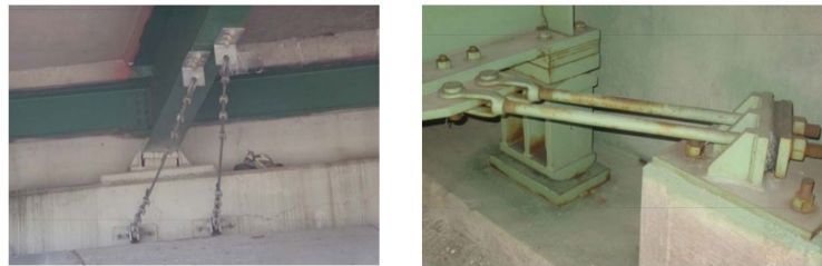
Figure E.3 Restrainer Cables (Left) and Restrainer Bars (Right) (Timothy et al., 2011)
