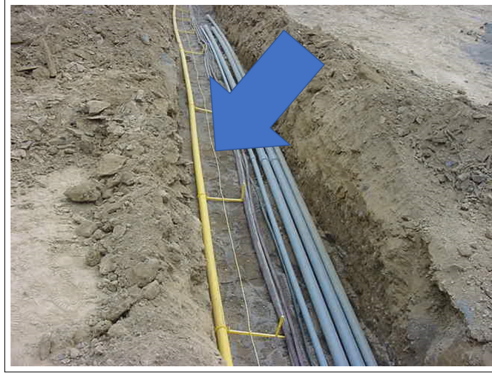
Figure 1.1: A tracer wire, noted by the arrow, used for locating multiple pipes. [34]
