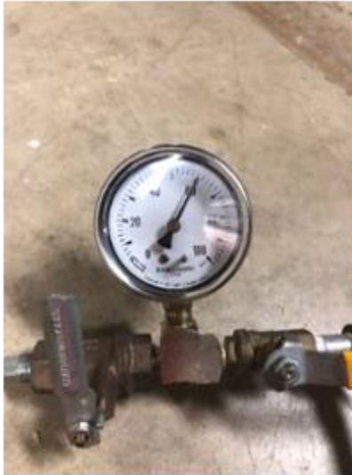
Figure 42 Pipeline Operating Pressure
