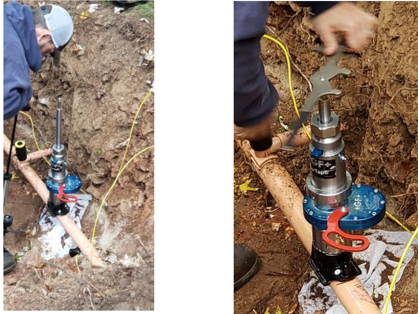
Figure 66 Hot Tap of Live Pressurized 2" Diameter Main
