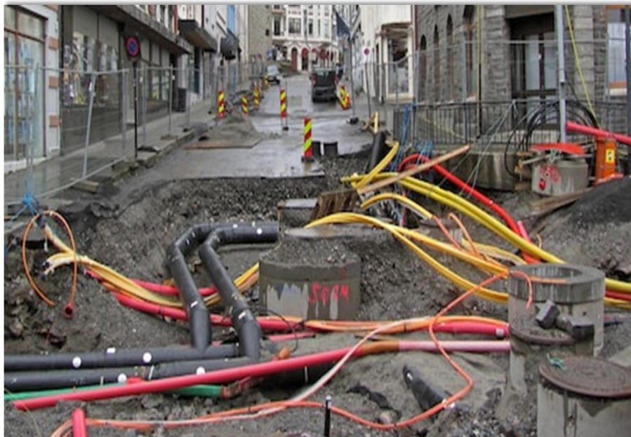
Figure 1 Example of Congested Underground Infrastructure
