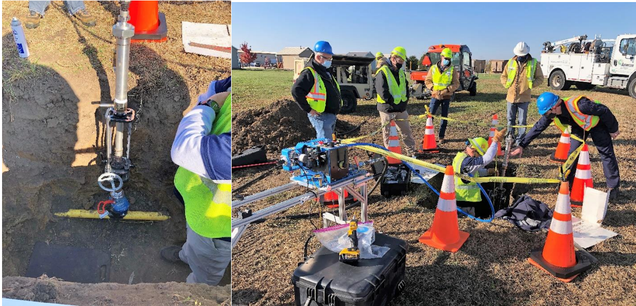
Figure 72 Live-Gas Insertion and Integrated Mapping System Operation
