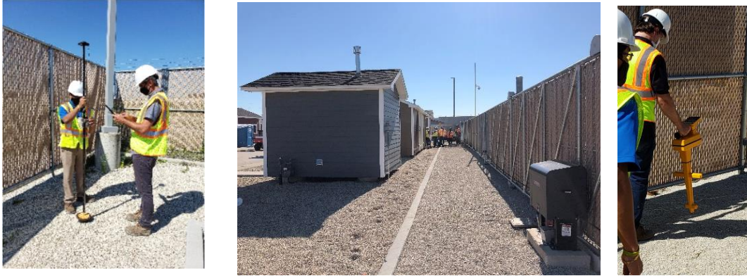
Figure 59 Collection of High Accuracy GPS Location along the Probe Path
