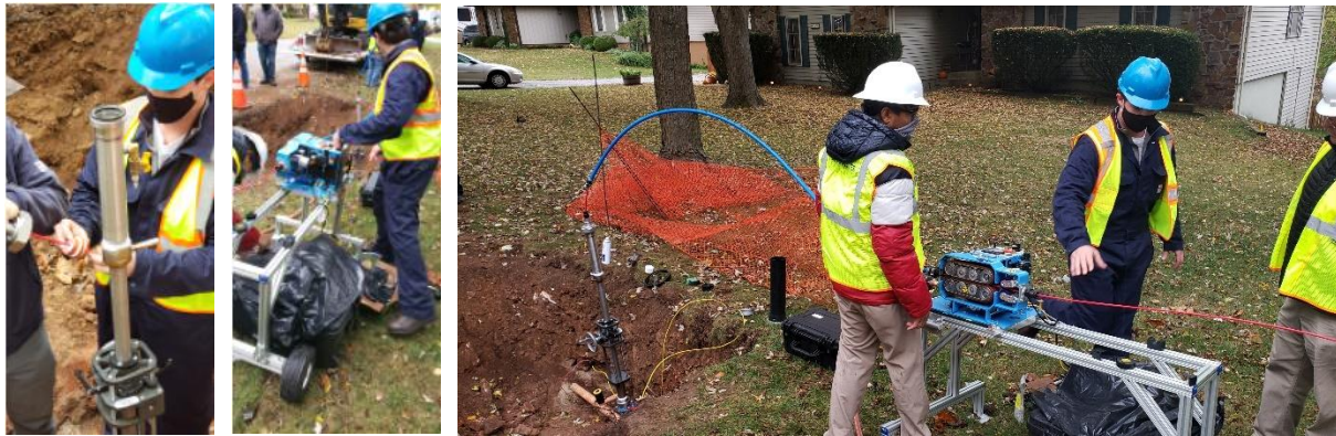
Figure 67 Insertion and Operation of the 3D Mapping Technology
