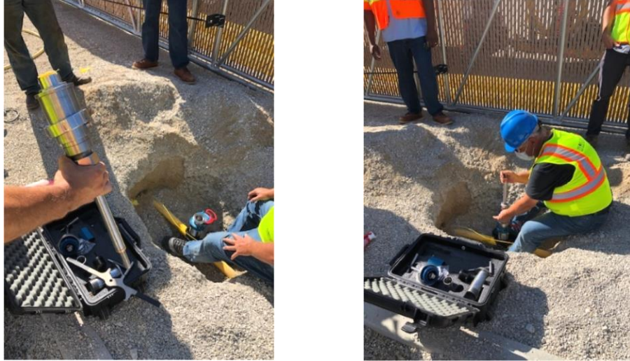
Figure 54 Hot Tap of Plastic Pipe for Live Natural Gas Mapping Launch
