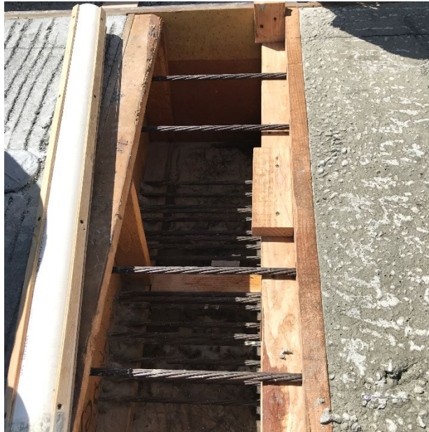
Figure 3.13 End Form Strand Setup
