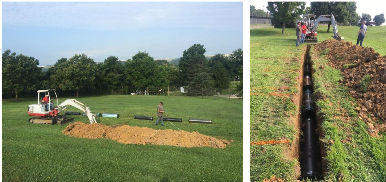
Figure 5-6: The pipe specimens being buried
