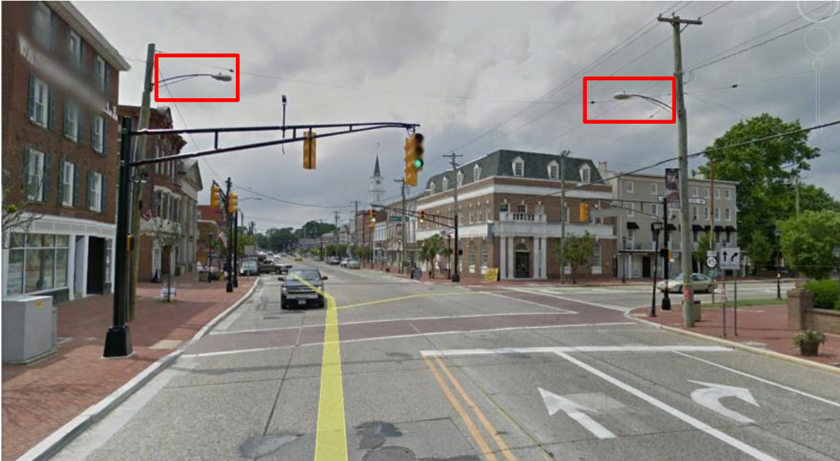
Figure 44: Presence of lighting in an intersection
