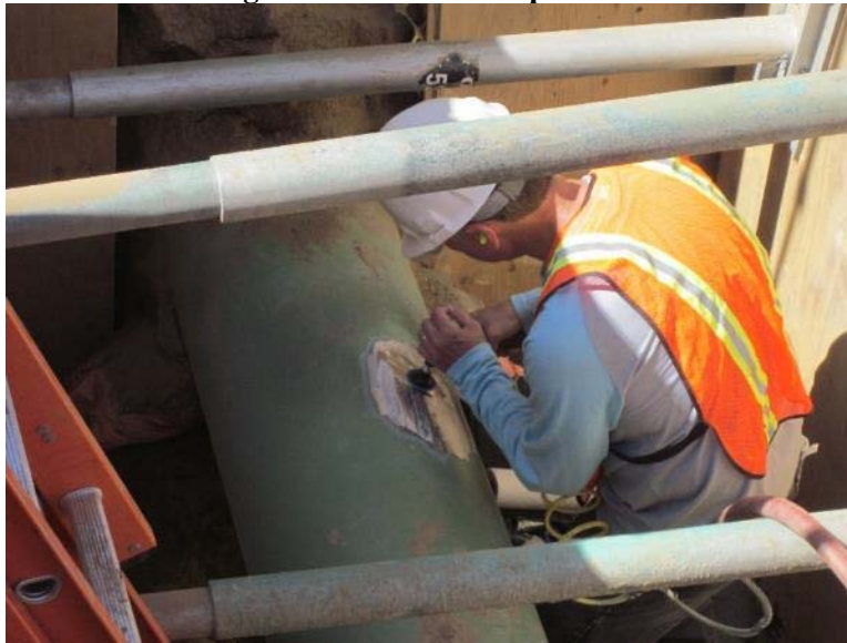
Figure 35: Surface Preparation
