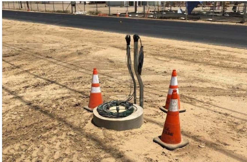
Figure 44: Footing and Conduit in Place
