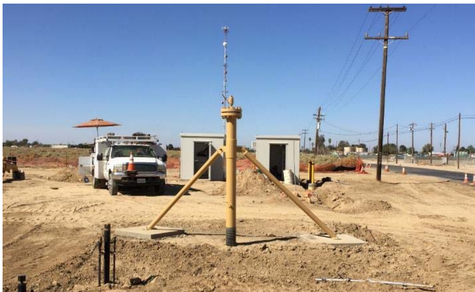
Figure 46: Equipment Sheds at Location 3 under Construction
