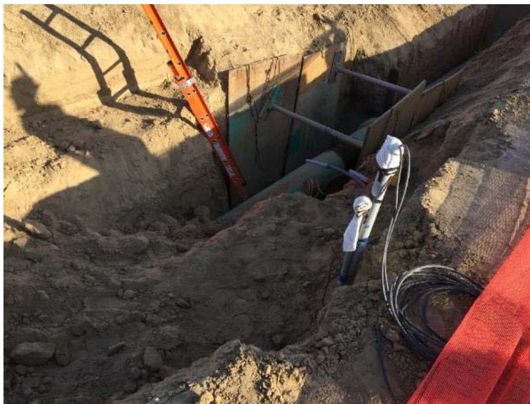
Figure 25. Excavation for Sensor Installation
