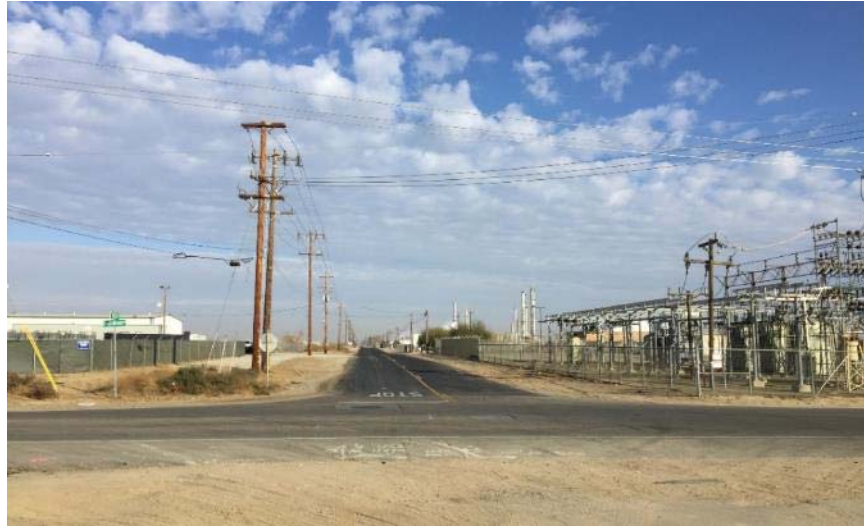
Figure 21. View of Utility Test Site
