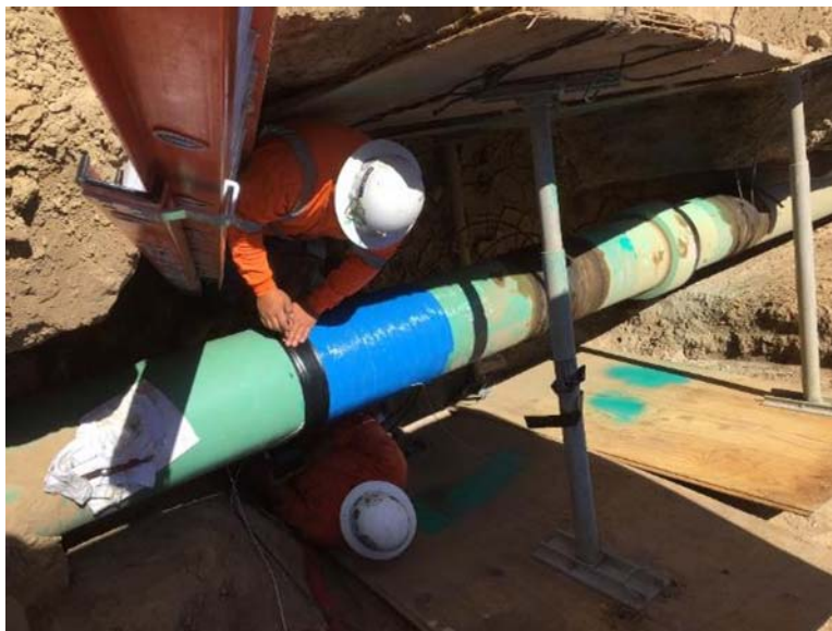
Figure 30. PVC Tape Wrap being applied over Viscotag Wrap
