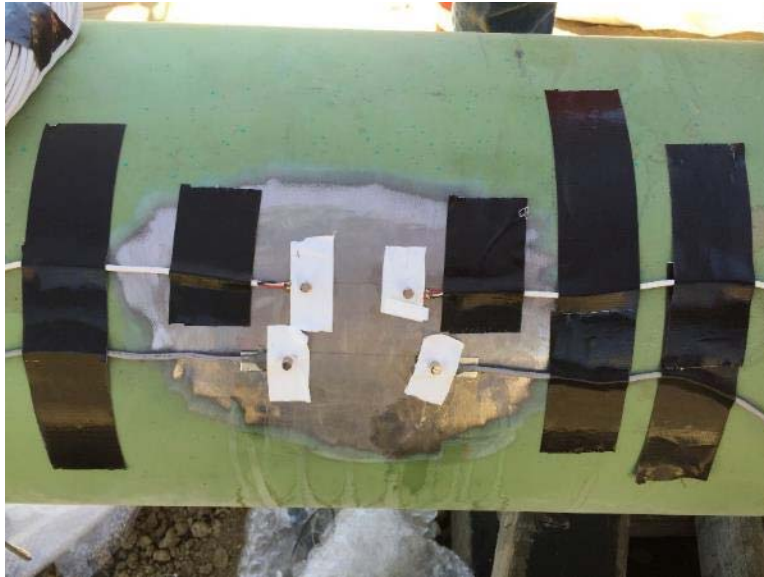
Figure 27. Sensors During Epoxy Cure
