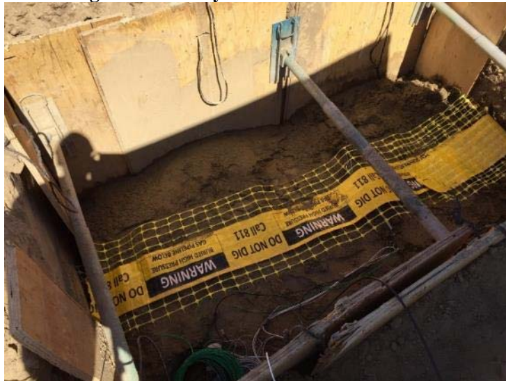
Figure 38: Slurry and Soil Sensors in Place
