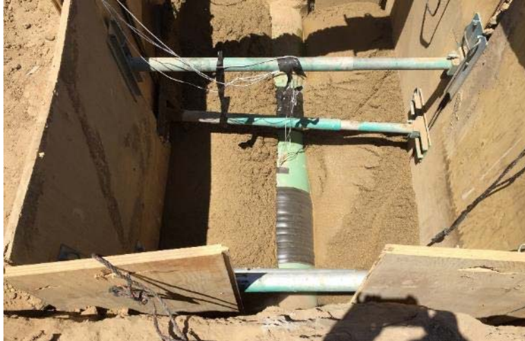
Figure 33. Excavation Partially Filled over Sensor Area
