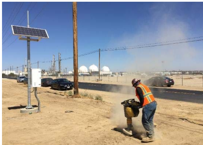
Figure 48: Compactor Testing
