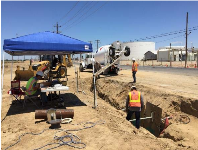
Figure 31. Monitoring Back Fill
