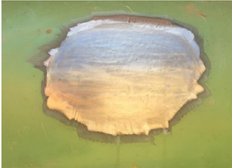
Figure 26. Cleaned Pipe Surface
