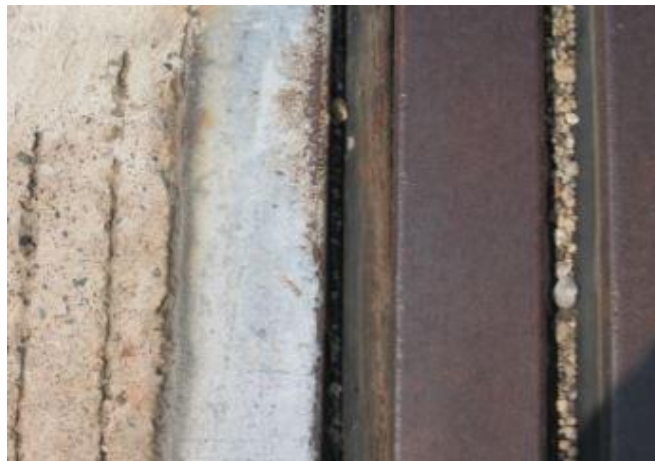
Figure 2.12. Modular joint with debris, preventing closure
