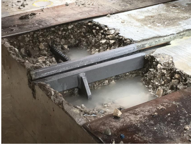
Figure 5.16. Hydrodemolition progress
