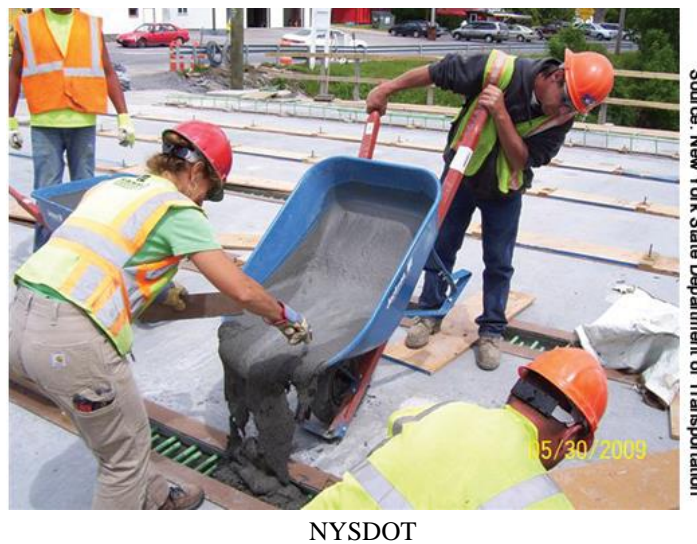
Figure 2.18. UHPC being place into a joint
