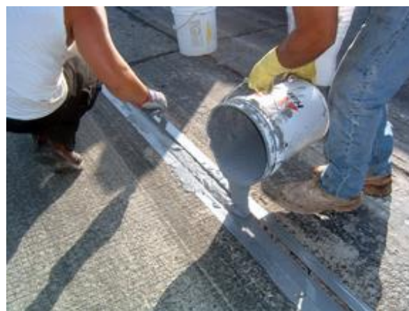
Figure 2.17. Elastomeric concrete for expansion joint repair
