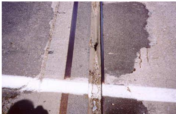
Figure 2.5. Strip seal joint with punctured gland
