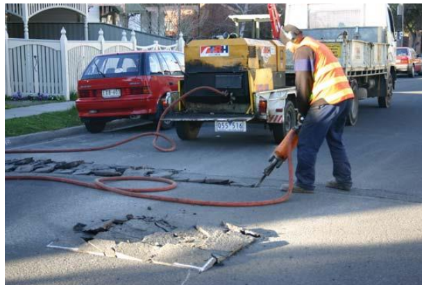
Figure 2.14. Pneumatic breaker
