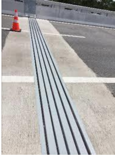
Figure 2.11. Typical modular joint
