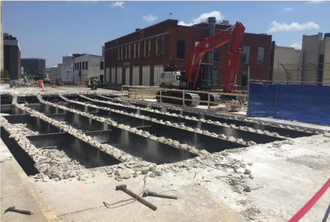
Figure 24. Staged deconstruction of the existing bridge in downtown Atlanta
