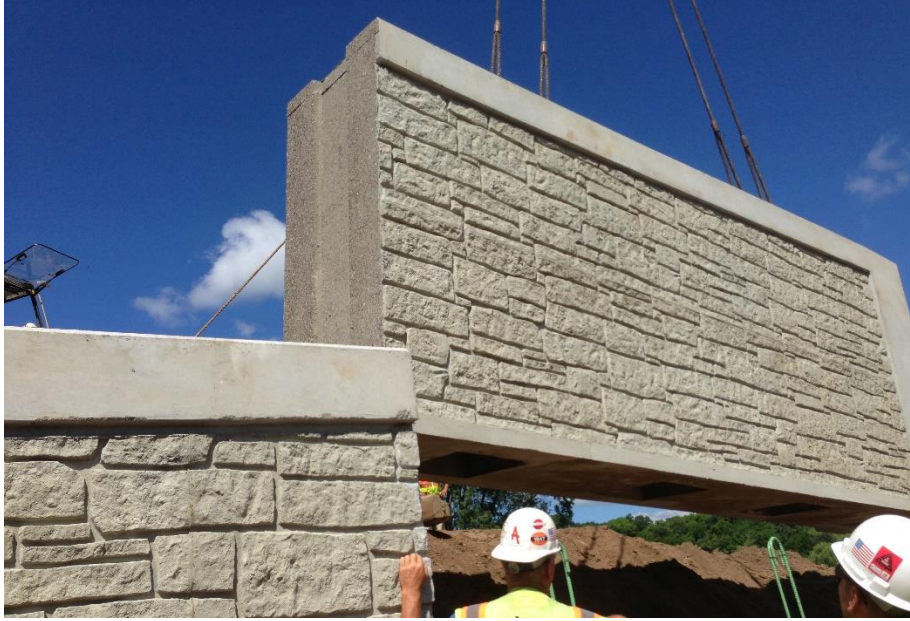
Figure 14. Precast abutment setting over piles with projecting, hooked, reinforcing steel bars
