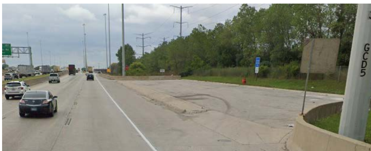
Figure 31. Example of Accident Investigation Site in Chicago (I-55 Exit 288 SB) (Source: Google Maps)
