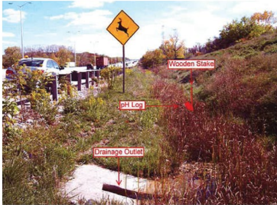
Figure 2.2: Localized Mitigation of High-pH Leachate from the Drain Near Receiving Waters using pH Log and Bioswale (Cavalline, 2018b)
