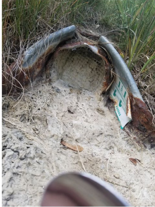
Figure 5.4 Underdrain Outlet at M53N-BRU-4 (RCCA Base, Year of Construction 2013, Age 7 years)
