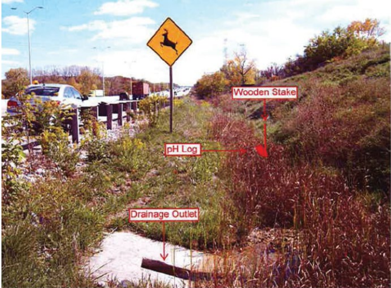
Figure 7.4 Localized Mitigation of High-pH Leachate from a Drain Near Receiving Waters using pH Log and Bioswale (Snyder, 2018)
