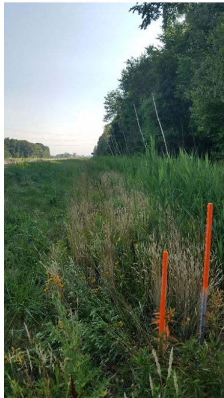
Figure 5.3 Underdrain Outlet at I94W-STC-2 (RCCA Base, Year of Construction 2010, Age 8 Years)
