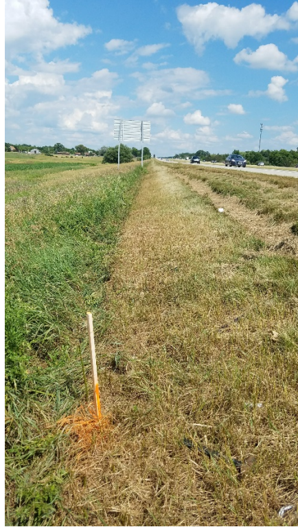
Figure 5.2 Underdrain Outlet I69W-Dav-1 (RCCA Base, Year of Construction 2010, Age 8 Years)
