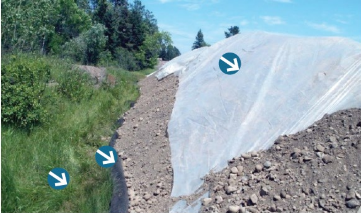
Figure 7.3 RCCA Stockpile Tarped with Plastic and Bounded by Perimeter Berm of Wrapped RCCA (Snyder, 2018)
