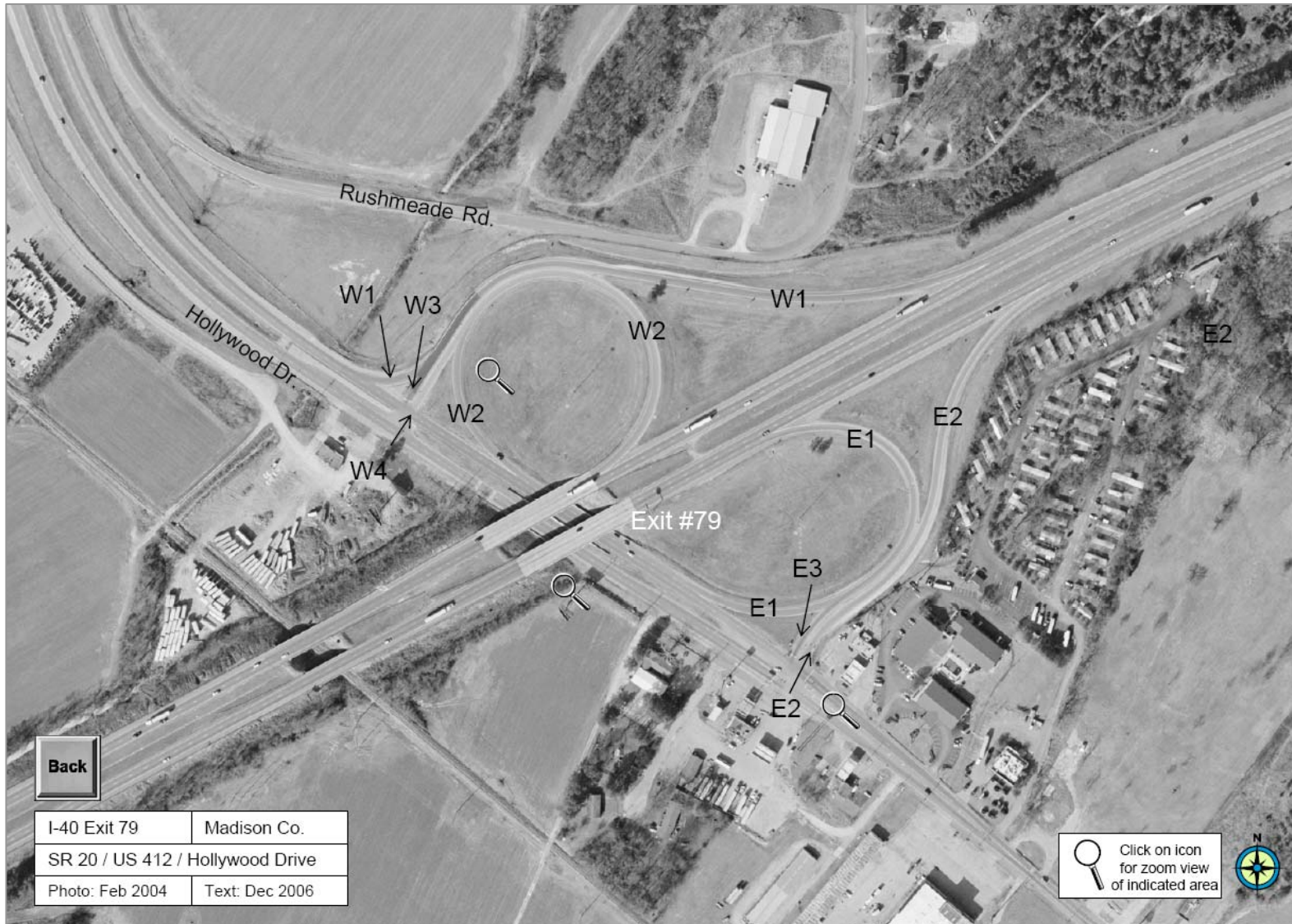
Figure 6. Example Interchange Photograph, Madison County
