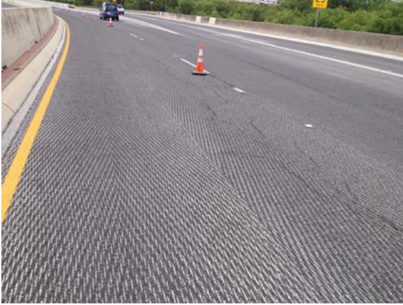
Figure 28. Photos taken from Wurzbach Parkway test site 3 months after the milling
