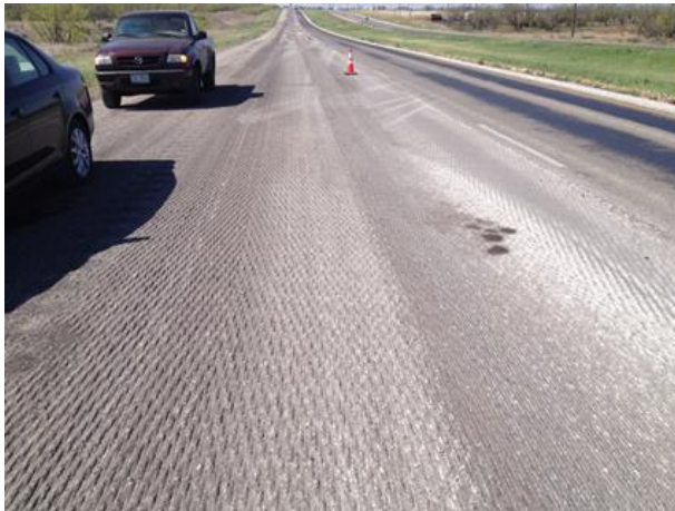
Figure 39. Photos taken from US 277 test site after the milling
