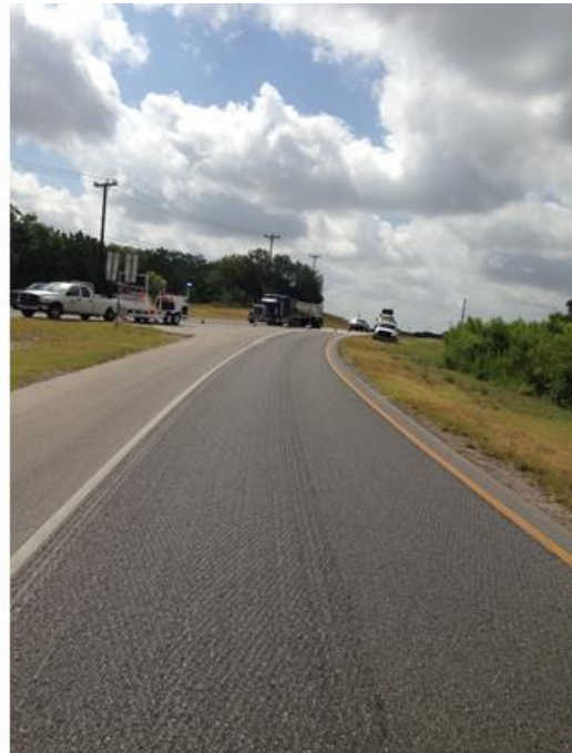
Figure 34. Photos taken from SH 151 test site 3 months after the milling
