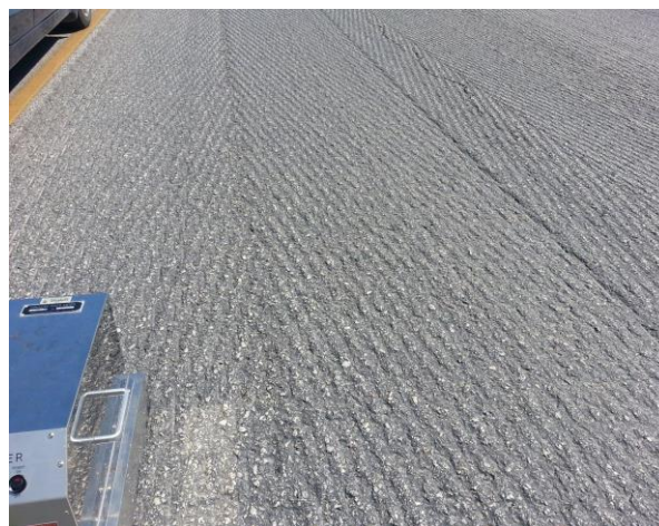
Figure 37. Photo taken from SH 151 test site 18 months after the milling
