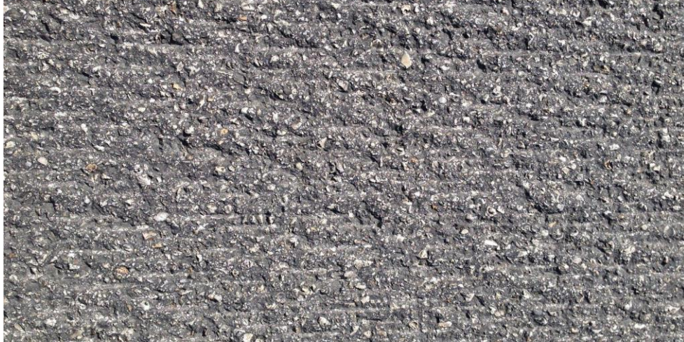
Figure 35. Photo taken from SH 151 test site 6 months after the milling
