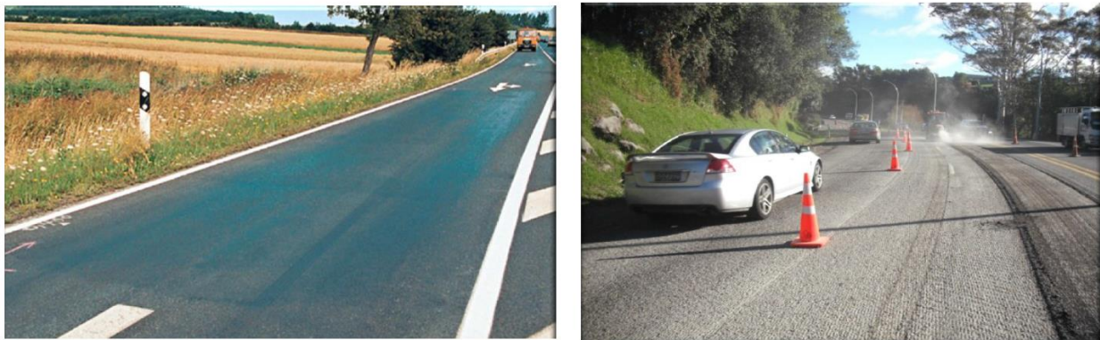
Figure 7. New Zealand Fine Milling Project: Before and After the Fine Milling
