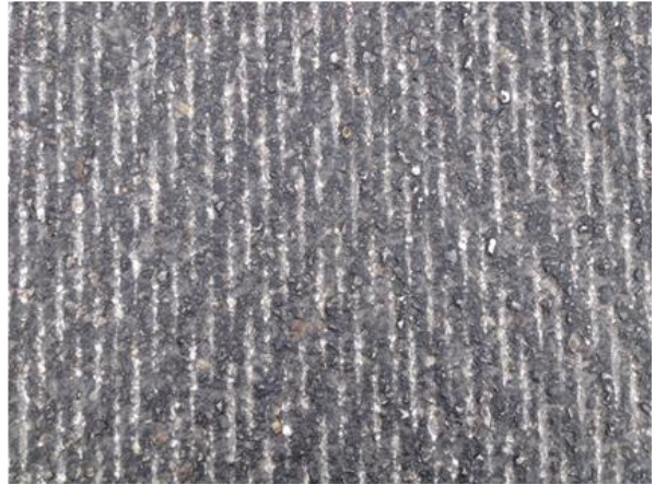
Figure 28. Photos taken from Wurzbach Parkway test site 3 months after the milling
