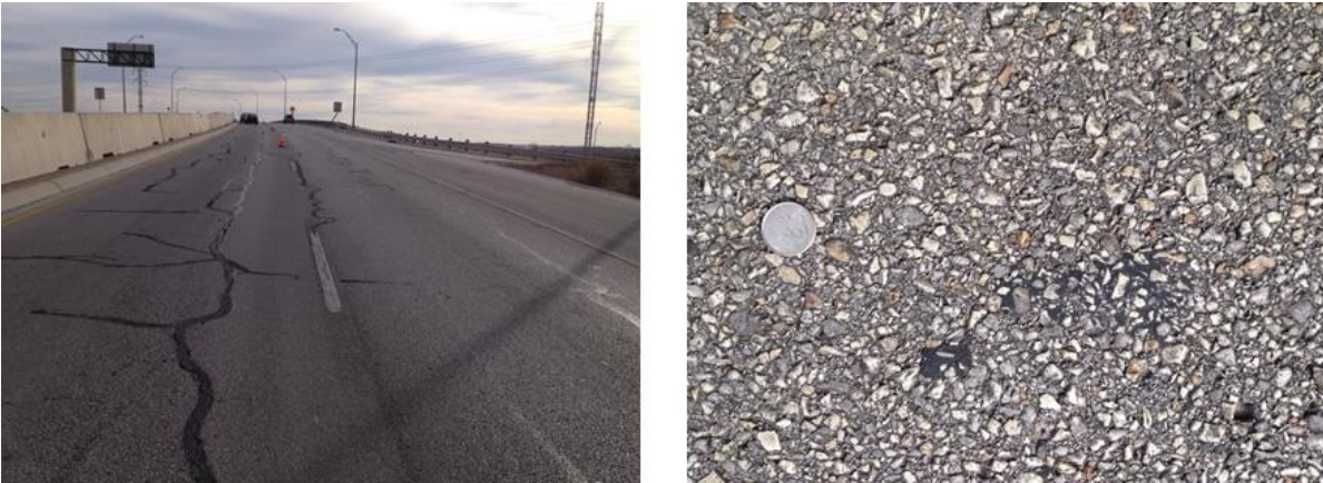
Figure 26. Photos taken from Wurzbach Parkway test site before the milling
