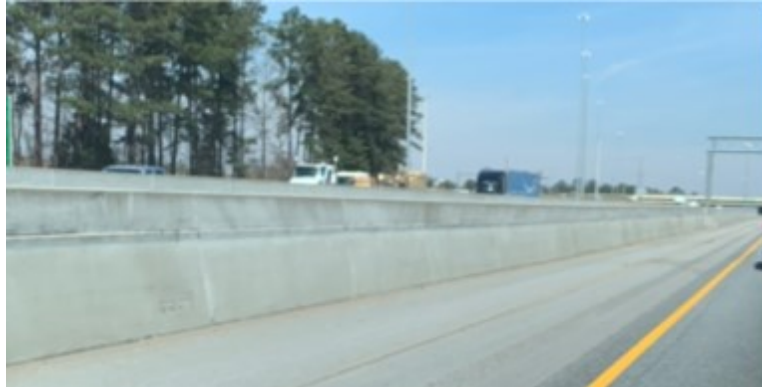
Figure 1. Example of a Concrete (rigid) Barrier.
