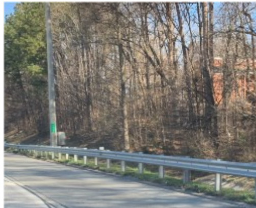
Figure 2. Example of a Guardrail with Steel Posts.
