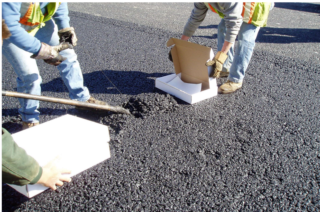
Figure 6. Sampling behind paver to obtain loose sample of asphalt mixture.
