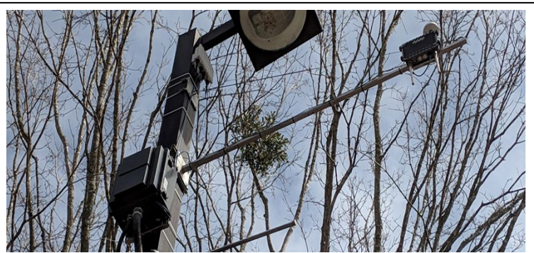
Figure 2: Edge node chassis (left), fiber to Ethernet (top), RSU (top right).
