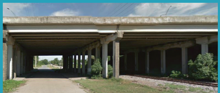
Figure 2: Underpass at the I-10 segment
