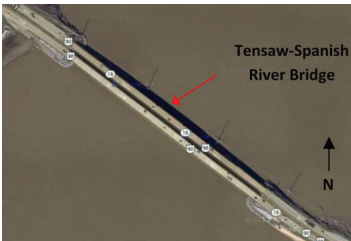
Figure 2: Aerial Image of the US 90/98 Tensaw-Spanish River Bridge
