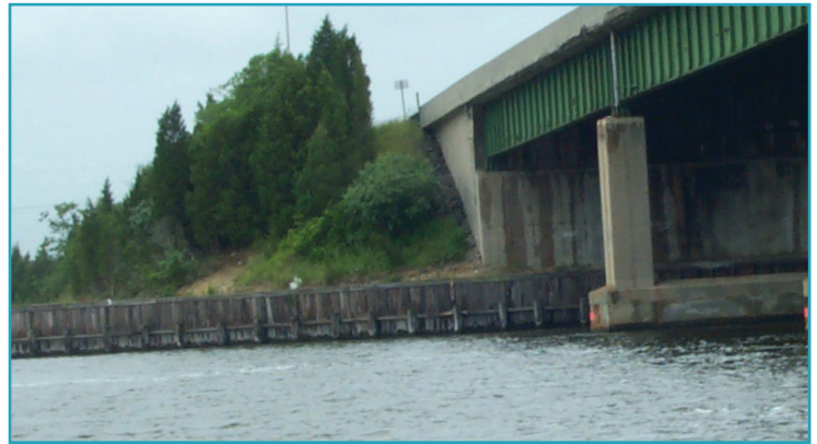
Figure 4: Example of typical timber bulkhead protection at a highway bridge abutment
