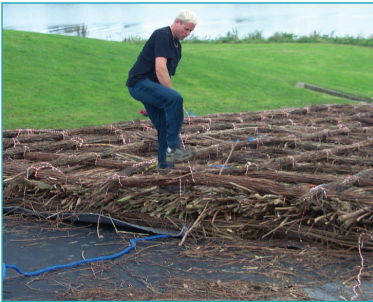
Figure 3: Representative willow mattress pad (assemble prior to submergence)
