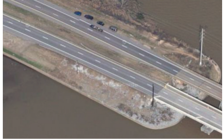
Figure 3: Oblique Aerial Image of the South Side of the US 90/98 Tensaw-Spanish River Bridge West Abutment. Source: Google Maps
