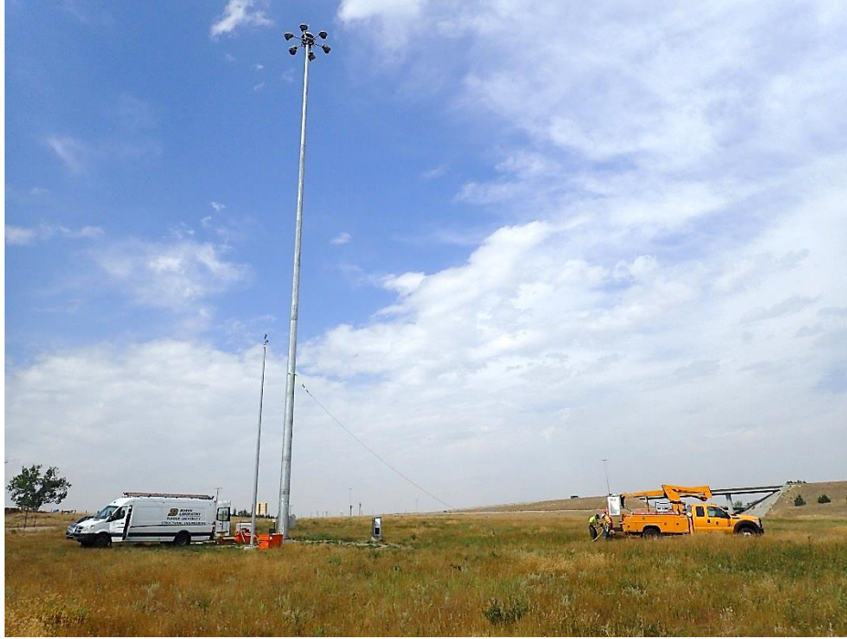
Figure 21. Pluck testing the HMLT at Buffalo Tri-Level
