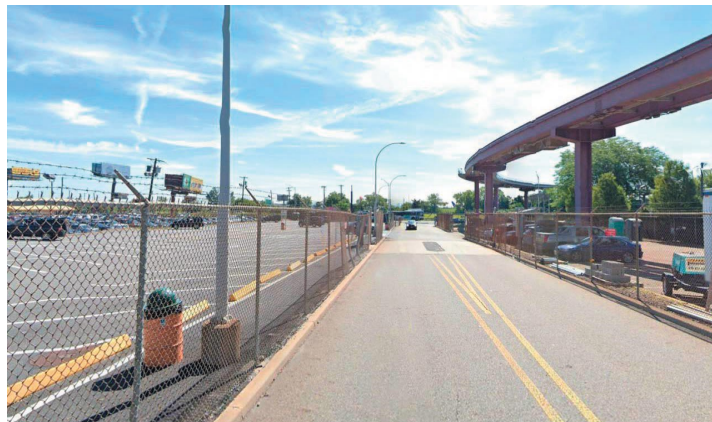
Figure 41. Land under the AirTrain tracks is currently used mostly for airport parking lots.
