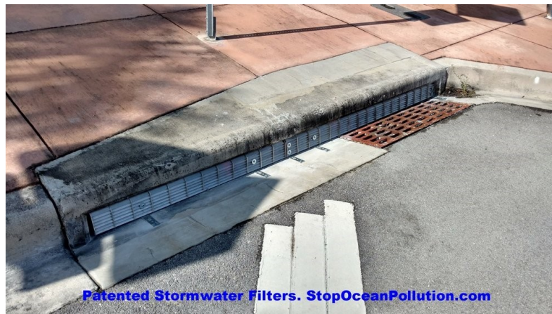
Figure 34. SOP Technologies' curb inlet filter
