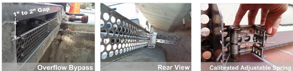
Figure 8. United Stormwater Automatic Retractable Screen
