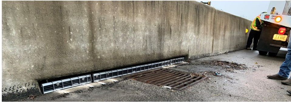
Figure 9. Installed screen on a median barrier inlet
