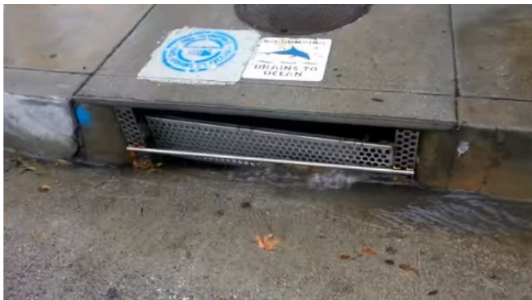
Figure 32. United Storm Water's Wing Gate ARS
