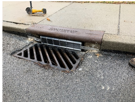
Figure 10. Installed screen on a curb inlet
