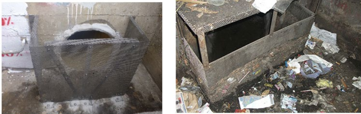
Figure 33. United Storm Water's connector pipe screen
