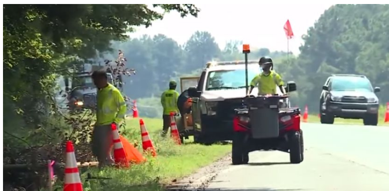
Figure 41. Use of all-terrain vehicles in roadside debris collection by ALDOT
