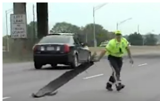
Figure 39. Manual removal of large debris from the roadway
