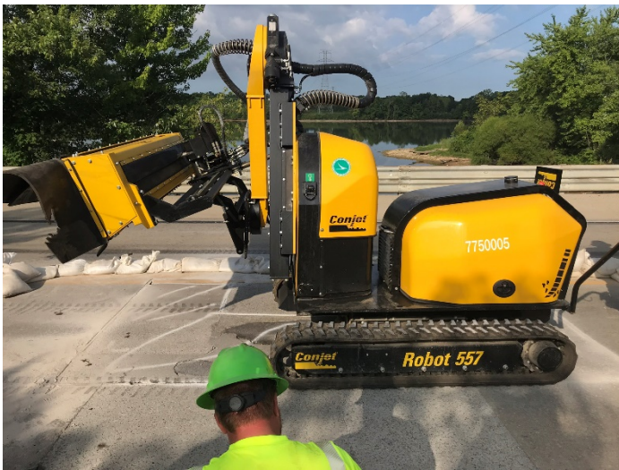
Figure 25: Deck Hydrodemolition on SR 257
