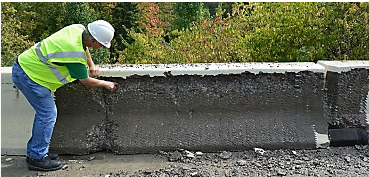
Figure 11: Interior parapet wall profile after hydrodemolition using the spray nozzle
