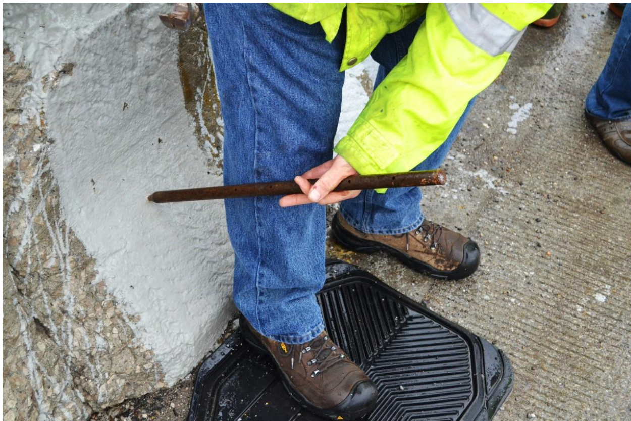
Figure 50: Impact test on parapets with stake and hammer
