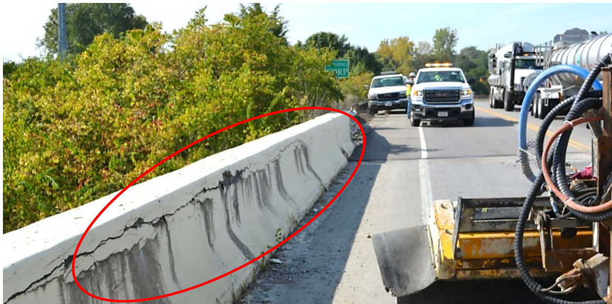
Figure 9: Parapet wall before hydrodemolition
