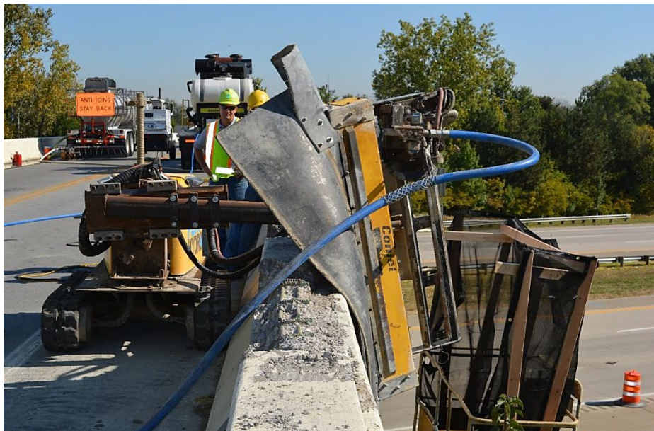
Figure 4: Hydrodemolition robot with articulated head for vertical surfaces
