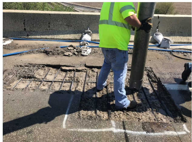
Figure 22: Hydrodemolition Training US-23 Bridge Deck
