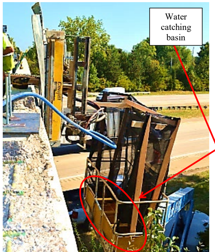
Figure 13: Water containment system for exterior parapet wall hydrodemolition
