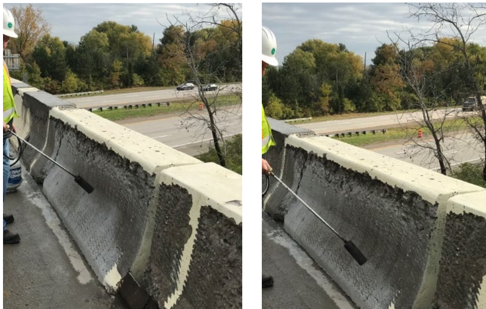
Figure 28: Drying the surface of the parapet walls
