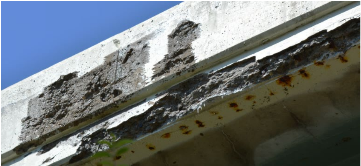
Figure 15: Exterior parapet wall profile after hydrodemolition
