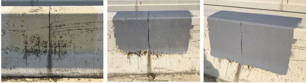
e) Product 3: Primer \xrightarrow{\hspace{10em}} Top Coat Figure 38: Photos of polyaspartic primer and top coat applications on SR142
