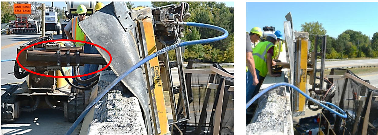
Figure 12: Exterior parapet wall hydrodemolition set-up
