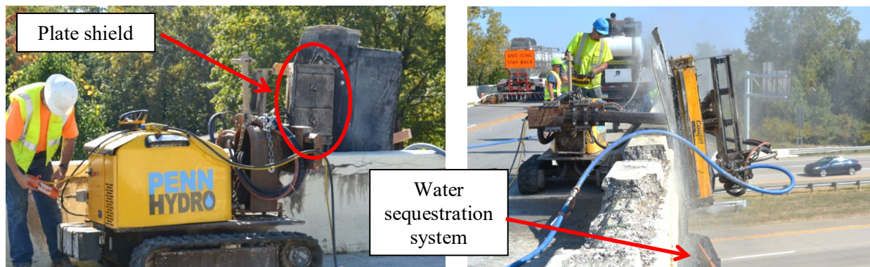
Figure 14: Exterior parapet wall hydrodemolition removal
