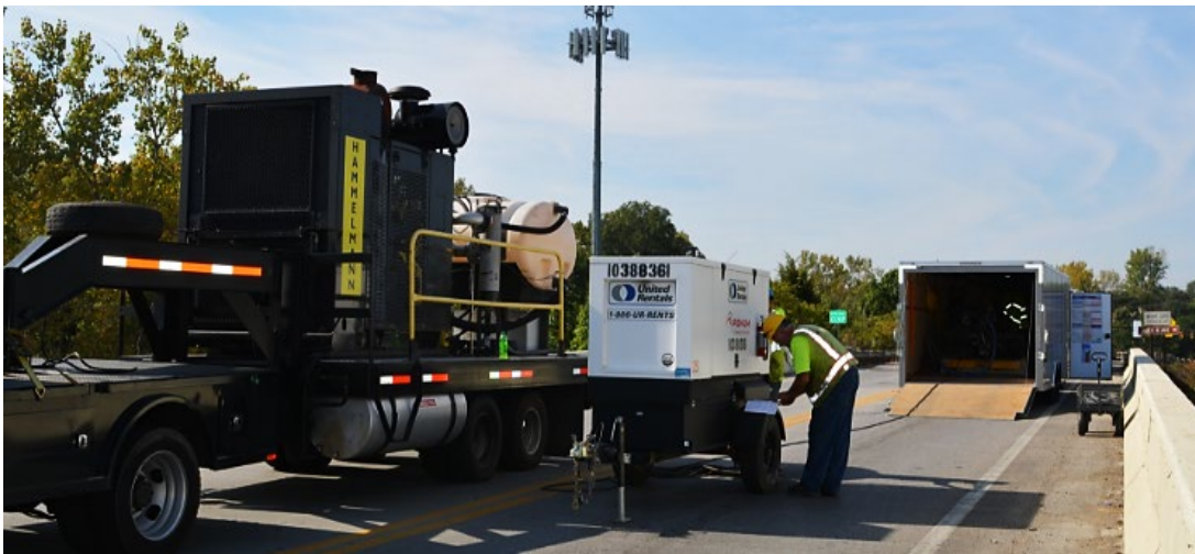
Figure 6: Hydrodemolition equipment setup
