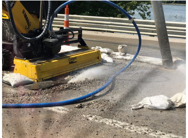
Figure 25: Deck Hydrodemolition on SR 257
