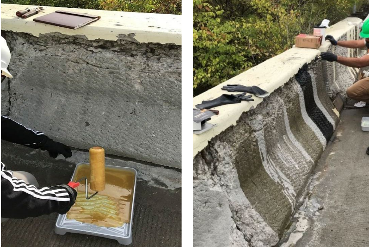
Figure 26: Rolling on of the primers of the polyaspartic products
