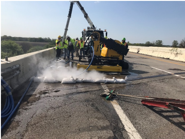
Figure 22: Hydrodemolition Training US-23 Bridge Deck
