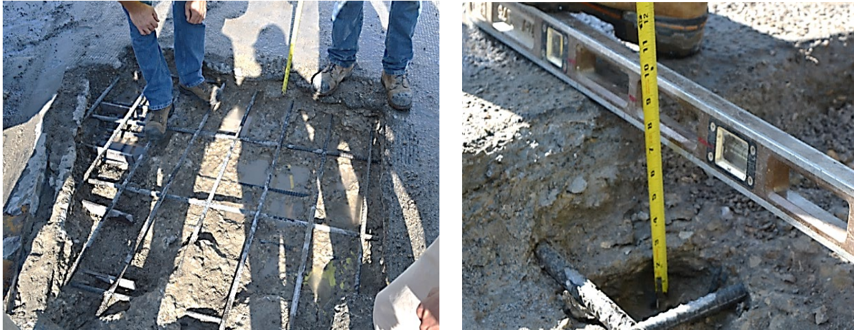
Figure 16: Hydrodemolition on the Gantz Rd. concrete bridge deck
