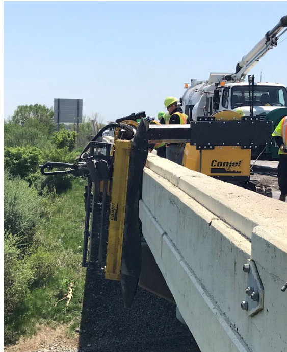
Figure 23: CONJET 557 Reaching over the Parapet Wall
