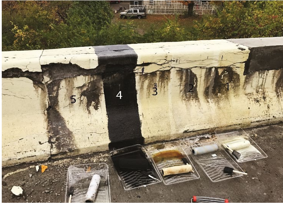
Figure 34: Application No. 2 of polyaspartic primer coatings
