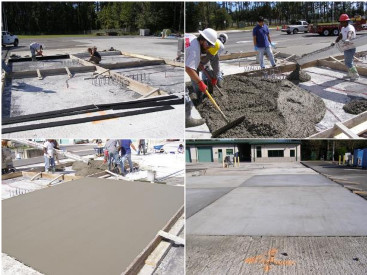
Fig 4.5 Construction of the slabs for Slab Study 1.
