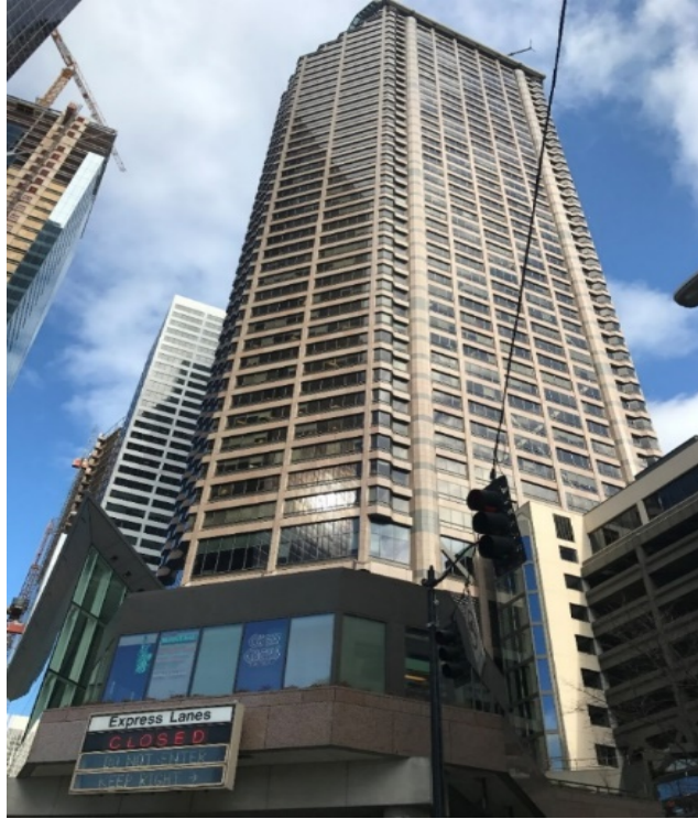
Figure 2.1 Seattle Municipal Tower
