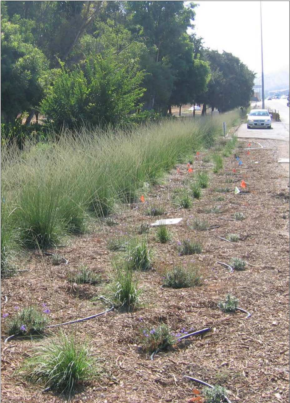
Transplants will need post-planting care. This planting in California has been mulched to suppress weeds and retain moisture and has drip irrigation to supply each plant with water during the establishment period. (Photograph courtesy Caltrans.)
