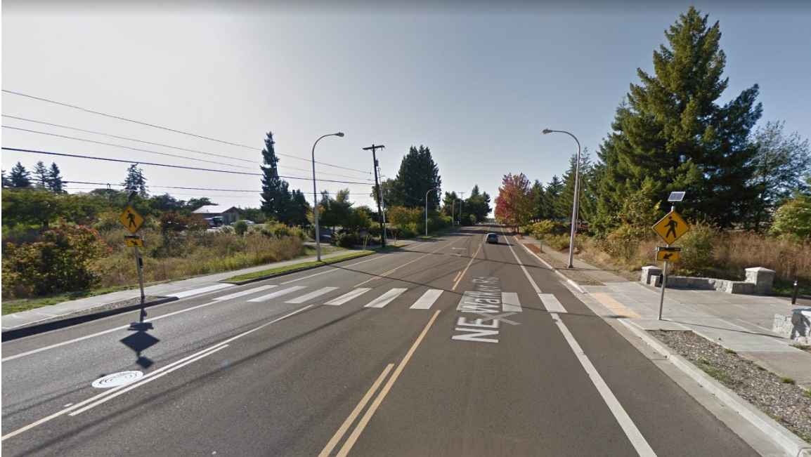
Figure 3.1: Category 1-NMR-OO: RRFB with no pedestrian refuge median island. Location: NE Walker Rd. Source: Google Maps (2019)
