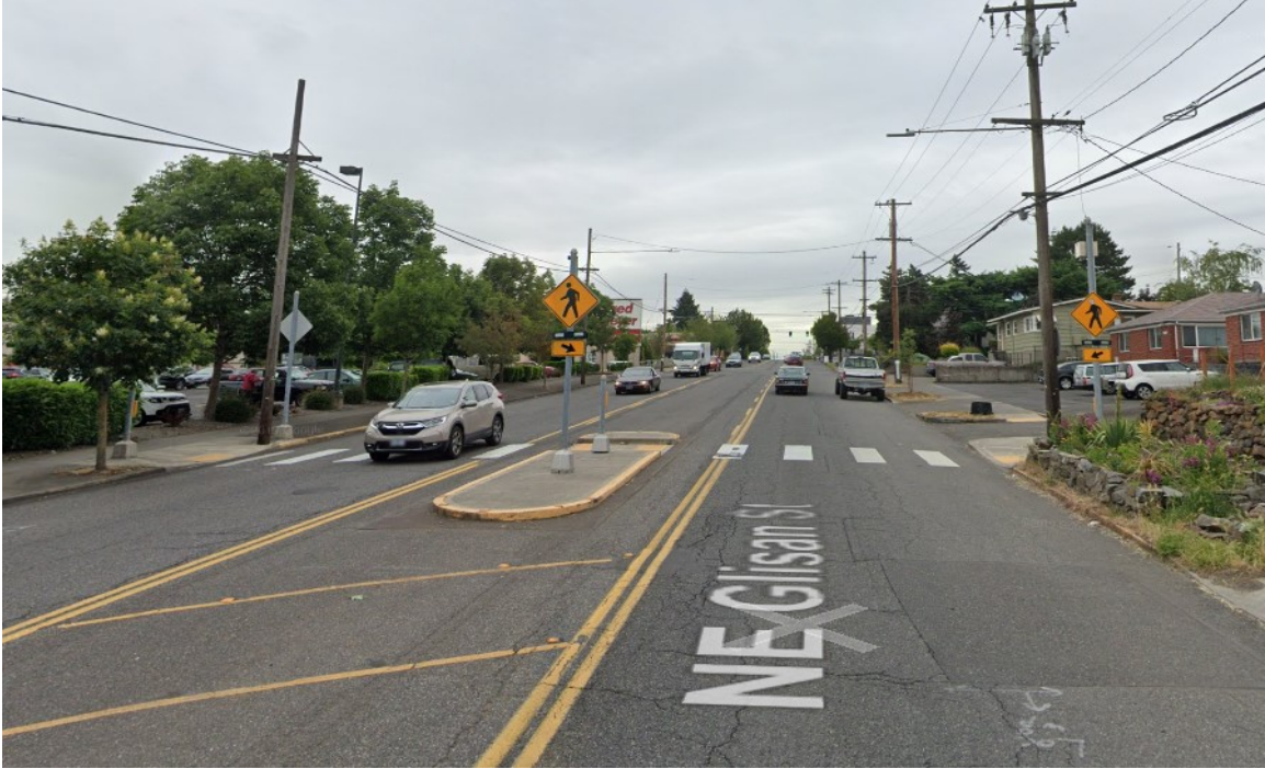
Figure 3.3: Category 3 MR-IO: RRFB with median island and median beacon. Location NE Glisan St. Source: Google Maps (2019)
