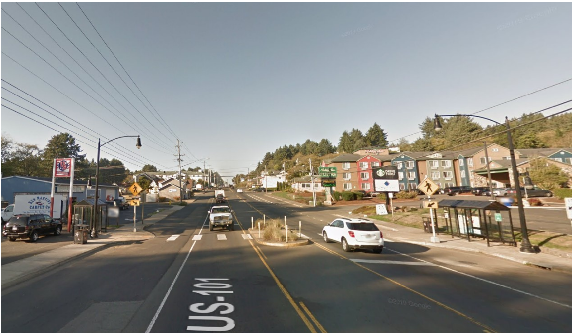
Figure 3.2: Category 2 MR-OO: RRFB with median island. Location US 101 in Lincoln City. Source: Google Maps (2019)
