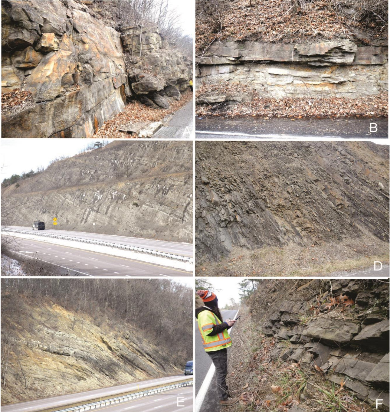
Figure 15. Stratification. A, Massive with stratification poorly discernible. B, Stratification horizontal. C, Stratification inclined parallel to road at < 45^\circ . D, Stratification inclined parallel to road, > 45^\circ angle. E, Stratification inclined into roadway. F, Stratification inclined away from roadway.
