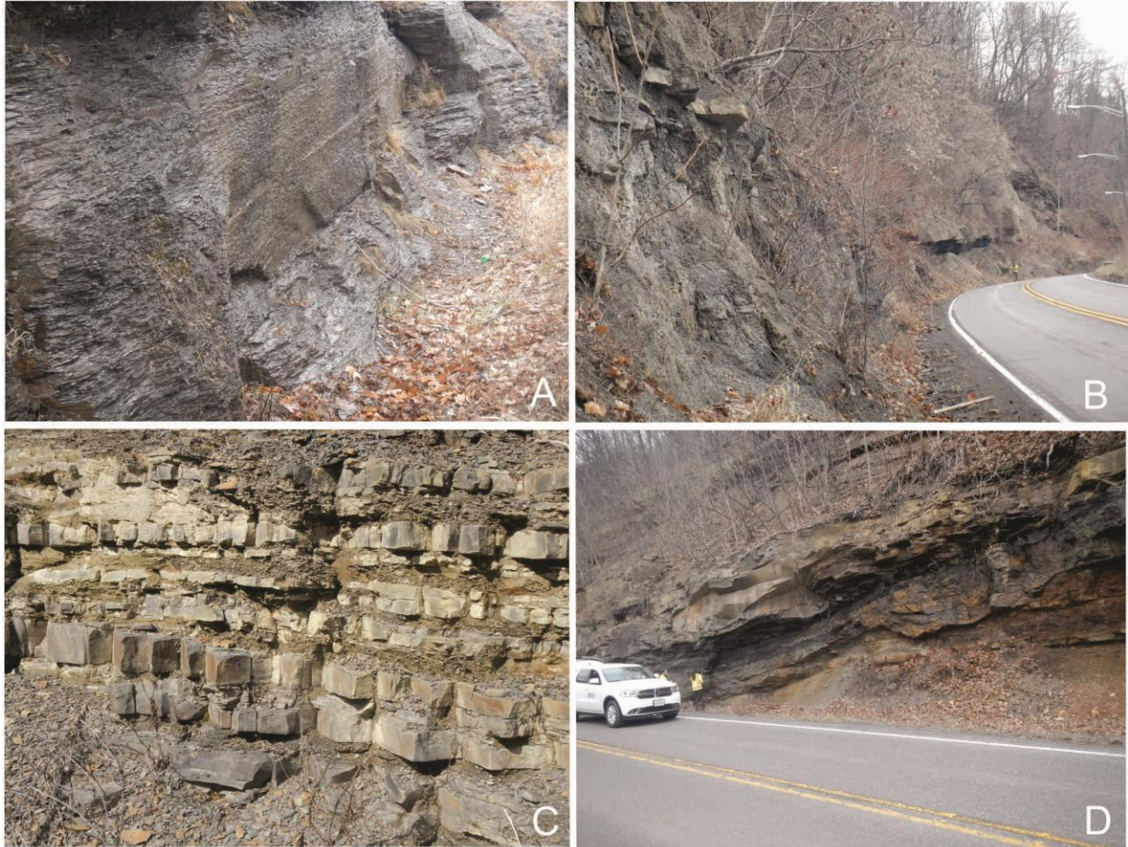
Figure 13. Differential erosion. A, Minor differential erosion within massive siltstone. B, Occasional differential erosion along sandstone interbeds. C, Many differential erosion surfaces within interbedded sandstone and shale. D, Major differential erosion at the contact between the Pottsville and Mauch Chunk formations.
