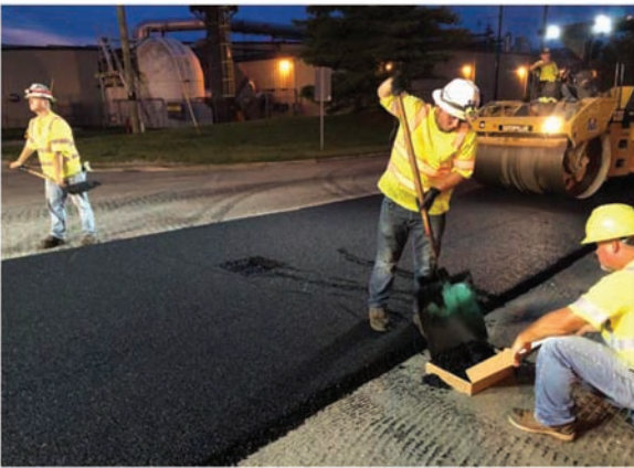
Figure 4.1 Sample collection at a Superpave 5 project site.
