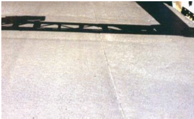
Figure 5.2 View of the formed joint behind the paver. After hand finishing, the joint becomes much less visible (Bergeron, 2004b).
