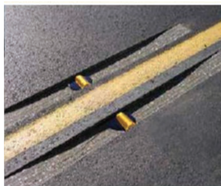
Figure 5.5 Installation of Banana Cut Marker (Dynatech, 2018).
