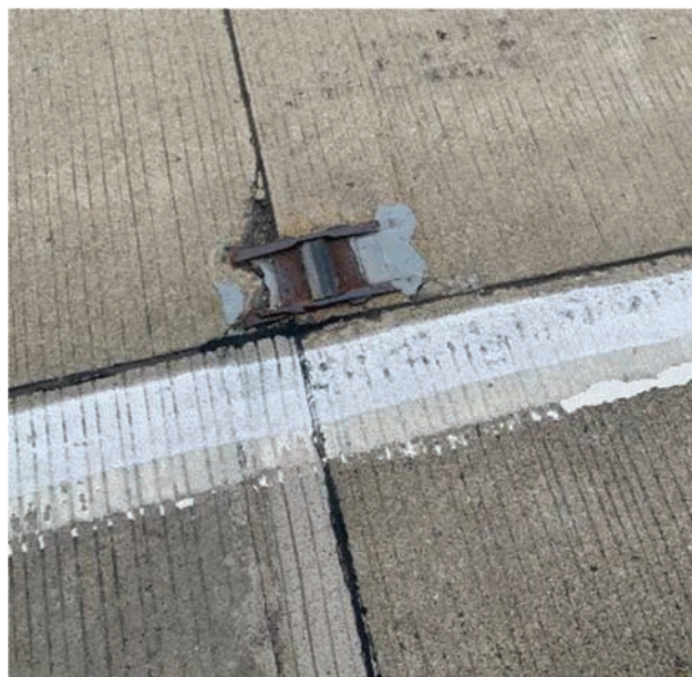
Figure 3.6 Damage to the longitudinal joints caused by RPMs (West Lafayette, IN-US 52).
