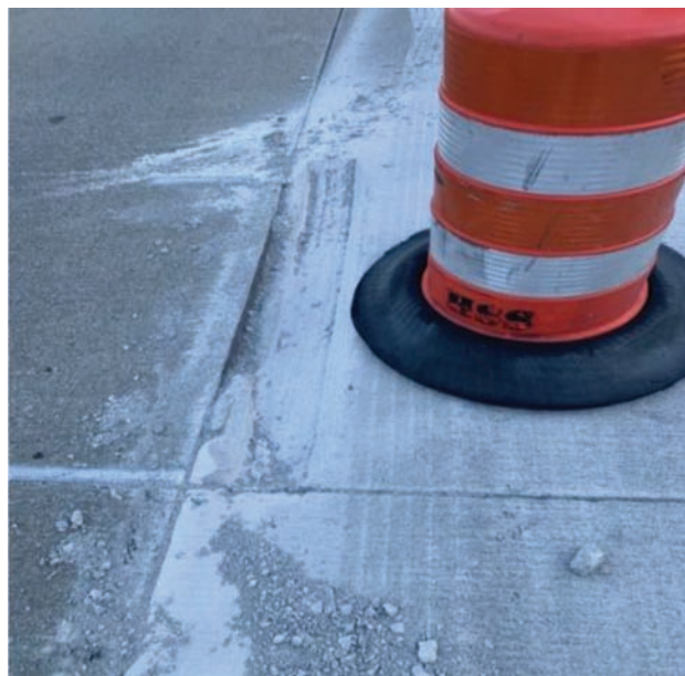
Figure 3.5 Damage to the longitudinal joints caused by removal of RPMs (Lafayette, IN-US 231).
