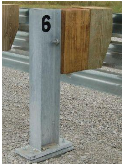
Figure 11. UBSP in Thrie-Beam Bullnose System [1]
