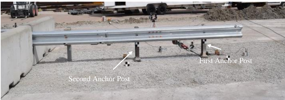
Figure 85. Test Setup, Test No. SPDA-1
