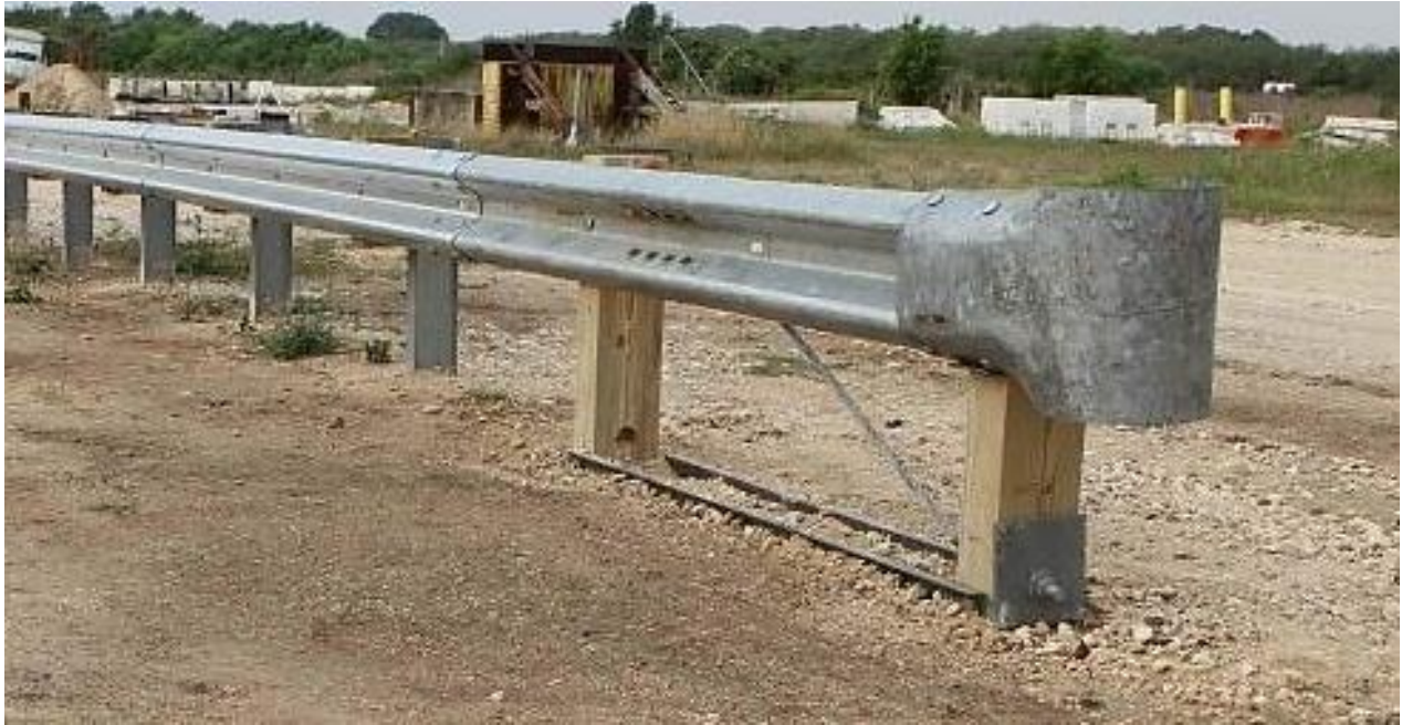
Figure 7. TxDOT Downstream W-beam Terminal [14]
