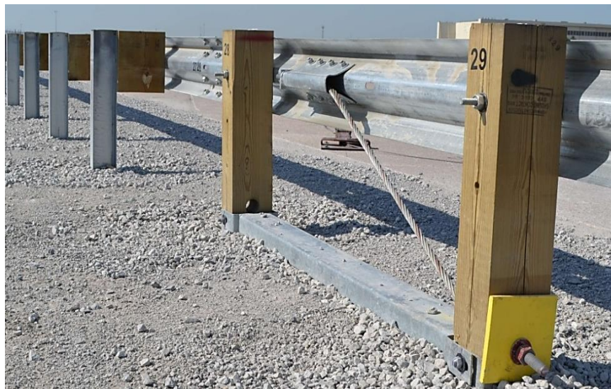
Figure 2. MGS Trailing-End, Guardrail Anchorage System [4]
