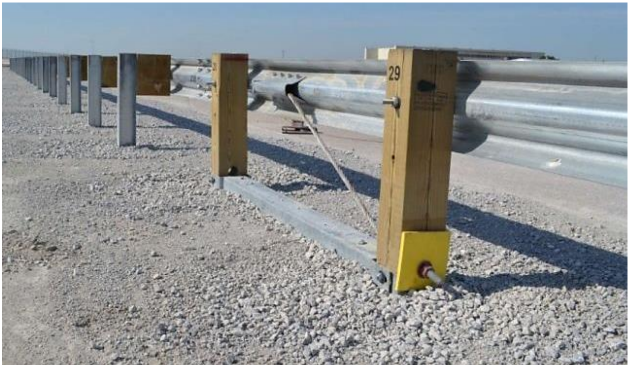
Figure 9. MGS Trailing-End Anchorage System [4]
