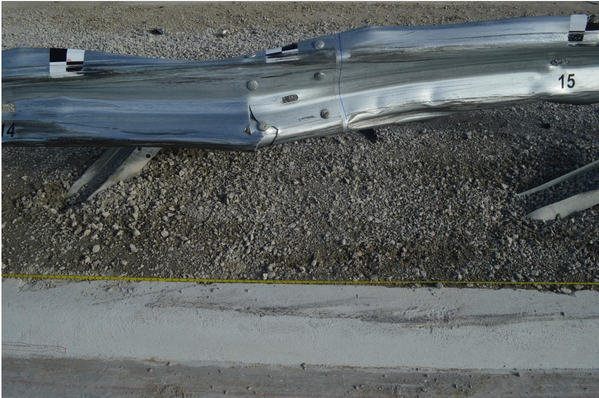
Figure 57. Curb Damage, Test No. MGSC-7
