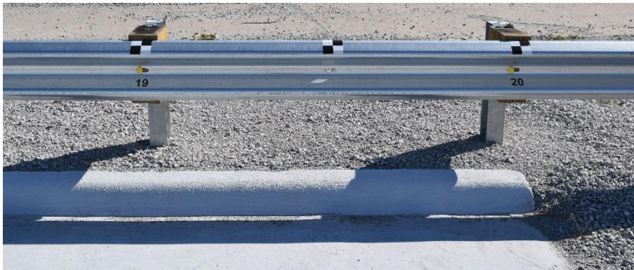
Figure 15. Test Installation Photographs, Test No. MGSC-7 20
