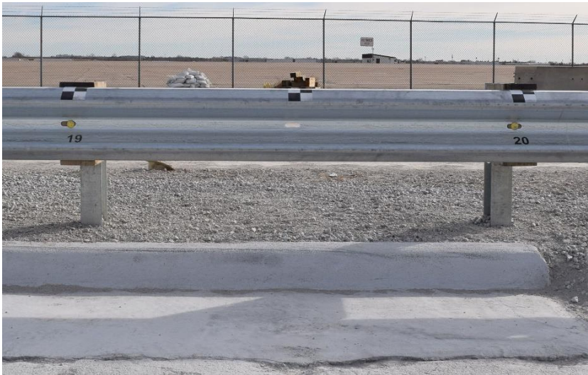
Figure 30. Test Installation Photographs, Test No. MGSC-8
