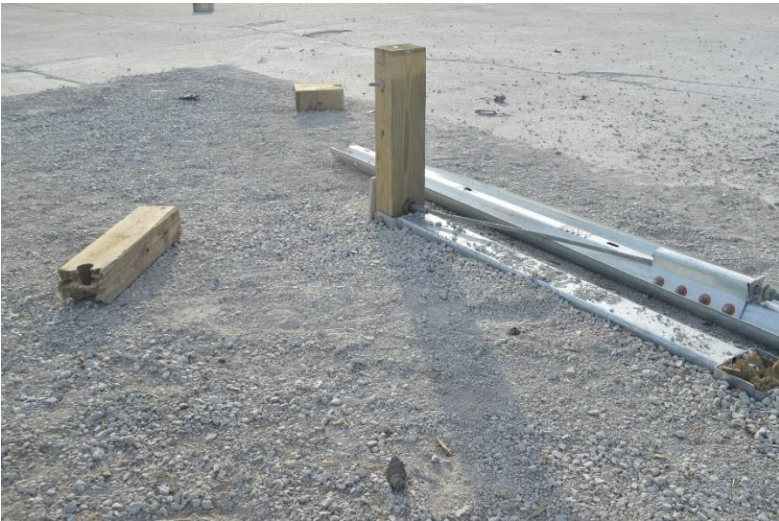
Figure 79. System Damage, Post Nos. 25 through 29, Test No. MGSC-8
