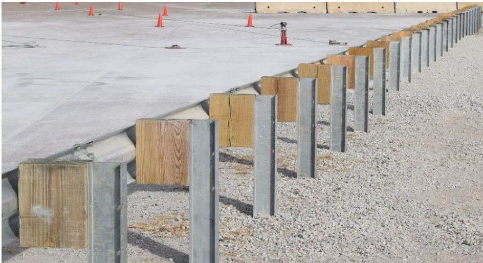
Figure 29. Test Installation Photographs, Test No. MGSC-8
