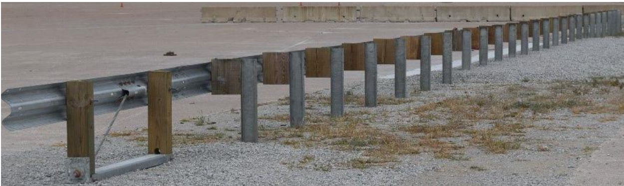
Figure 14. Test Installation Photographs, Test No. MGSC-7
