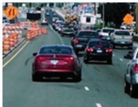
(f) Traffic can cause hazards for bridge inspection team and motoring public (Oregon DOT, n.d.)
