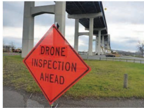
Figure 6.7 Drone inspection warning sign for motorists (Zink, 2015).
