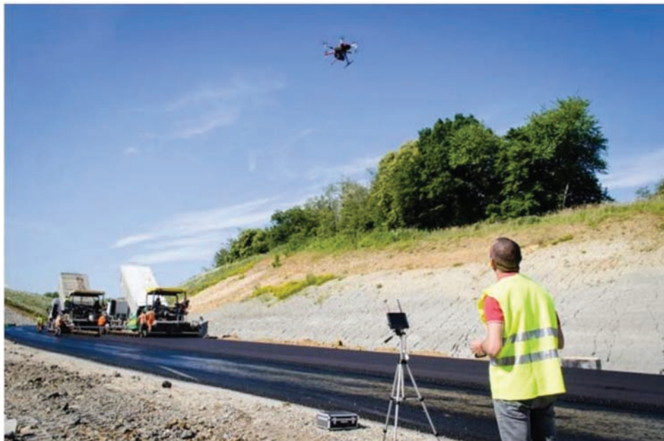
Figure 6.13 Construction progress and inspection (Winfield, 2018).
