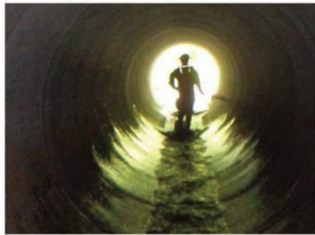
(a) Confined spaces (Edwards Diving Services, n.d.)
