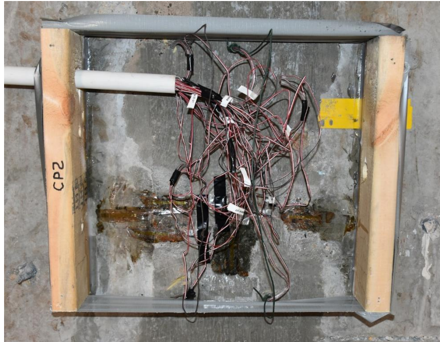
Figure 51. Closure Pour 2 high resolution picture during static loading of Load Test 1.2.
