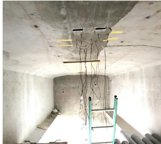
Figure 13. Closure pour with rebar gages installed.
