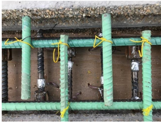
Figure 11. Closure pour prepared for concrete placement.
