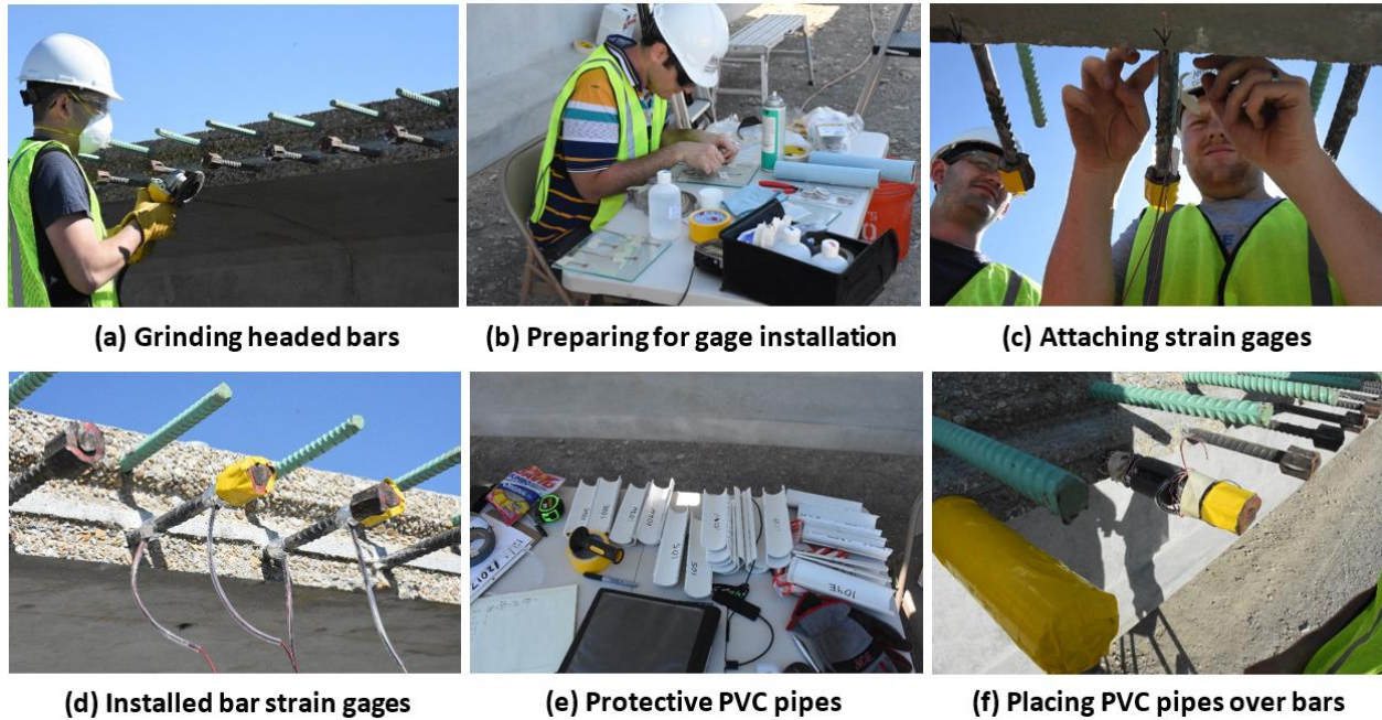
Figure 6. Strain gage installation at Forterra Structural Precast plant in Caldwell, Idaho.
