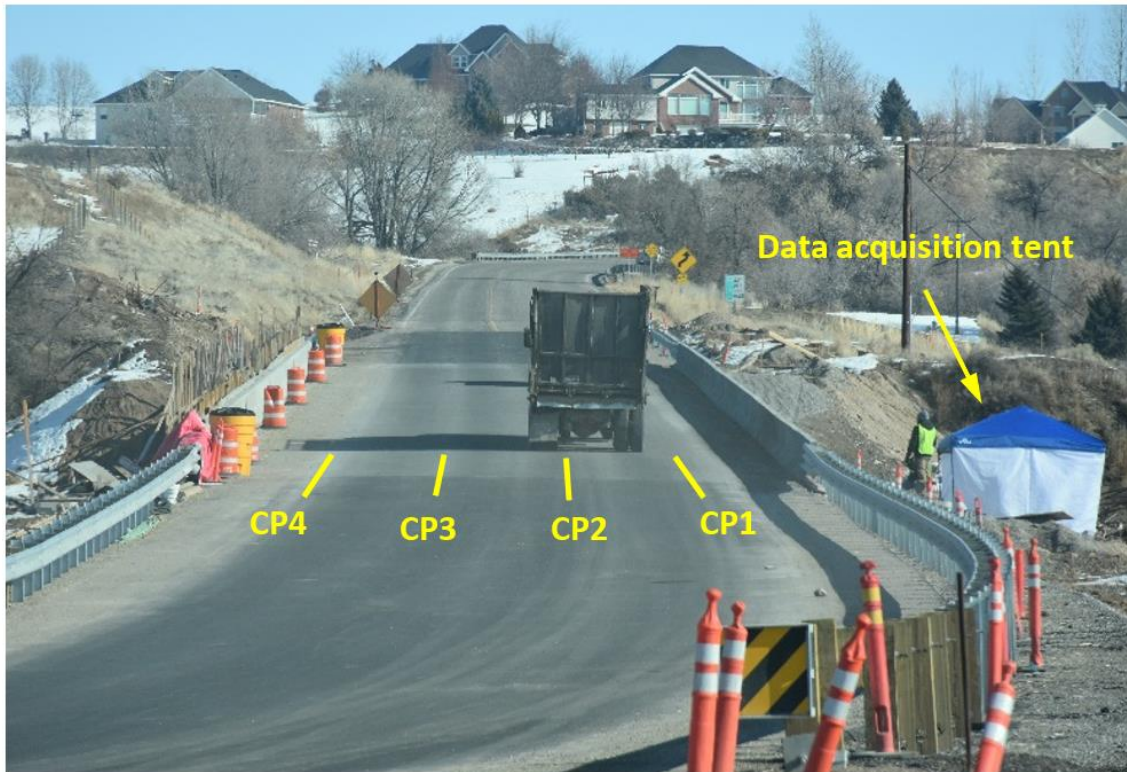
Figure 35. A three-axle truck traveling over the bridge.
