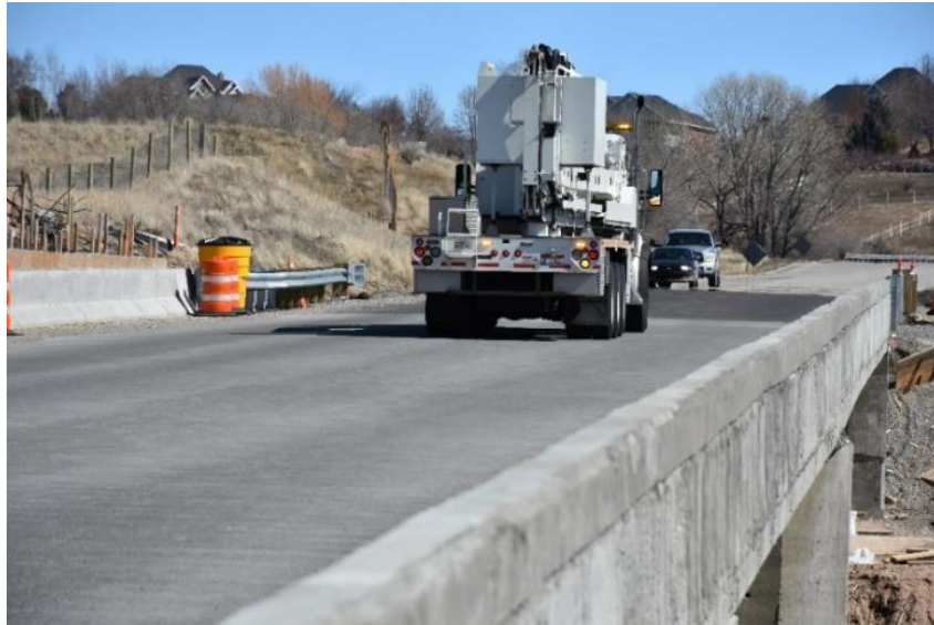
Figure 33. Large UBIT dynamic test.
