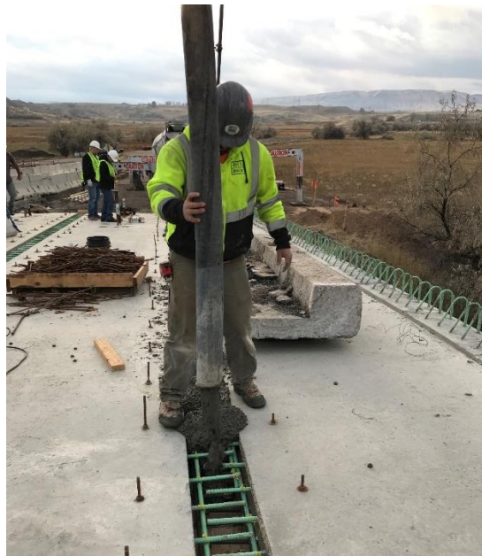
Figure 12. Placement of concrete in closure pour.
