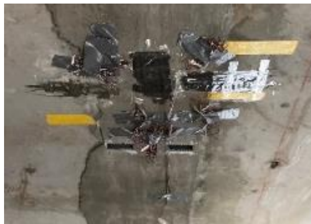
Figure 17. Filling pores on concrete surface with epoxy.
