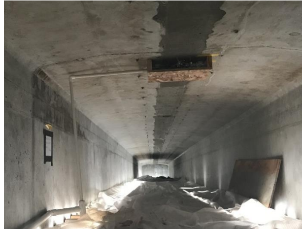
Figure 21. PVC conduit protection for strain gage wires.
