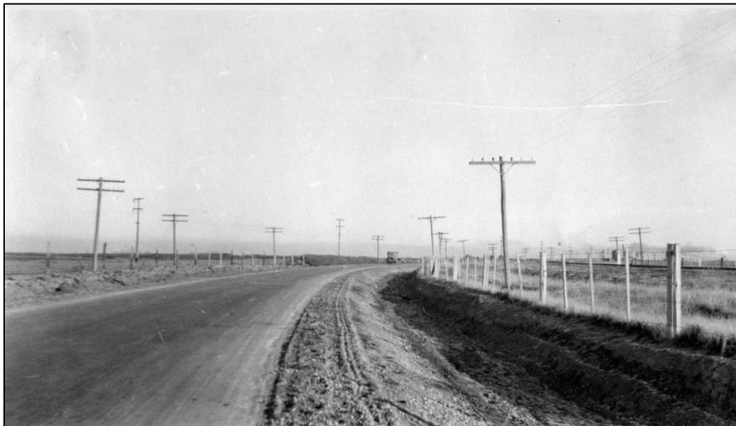
Figure 32. Typical highway construction on the Yellowstone Park Highway in Bingham County in 1923 showing an early type of bituminous surface treatment, 18-foot roadway, gravel shoulders, and ditches. 198
