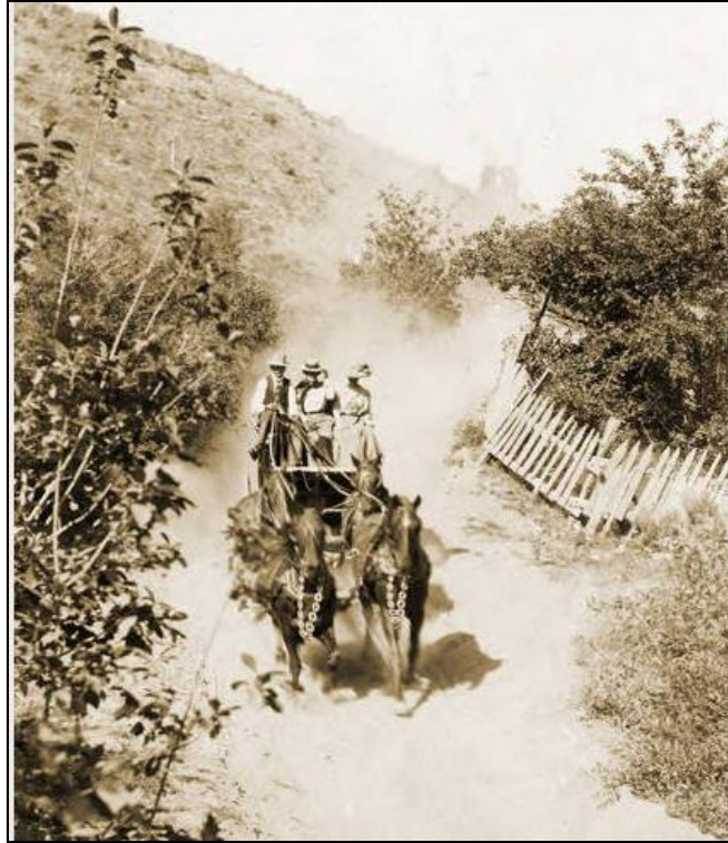
Figure 9. Stagecoach on toll road to Idaho City, 1904. 75
