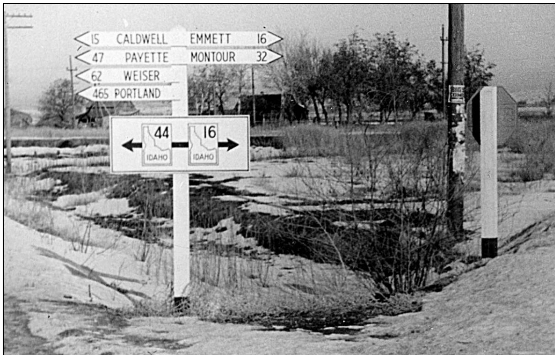
Figure 48. Typical 1930s informative and directional signage. 276
