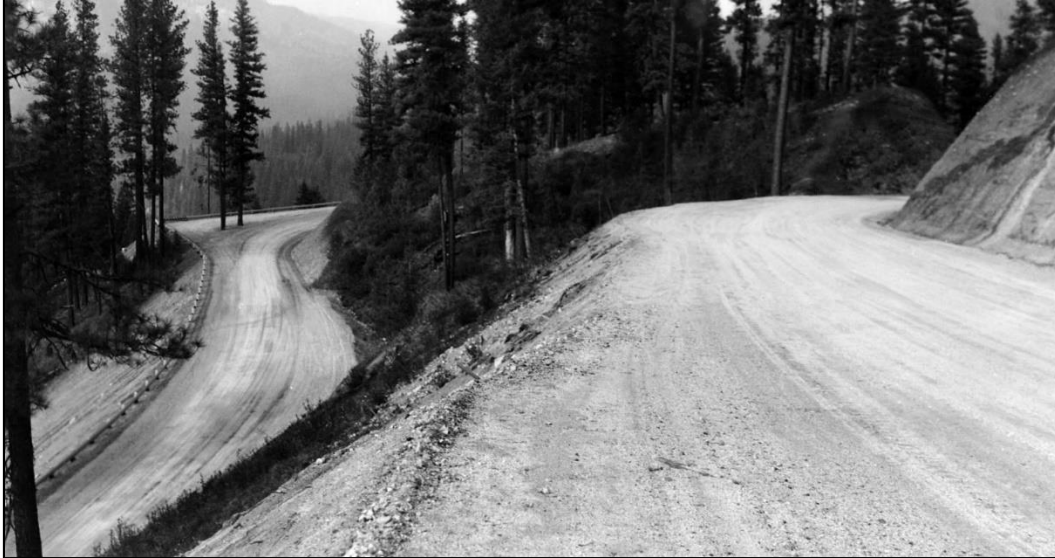
Figure 43. New construction on Idaho City-Stanley Forest Highway between Idaho City and Lowman in 1939 shows roadway design incorporating new concepts, including new Tuthill guardrail and roadside parking area at top left with mature trees preserved. 269
