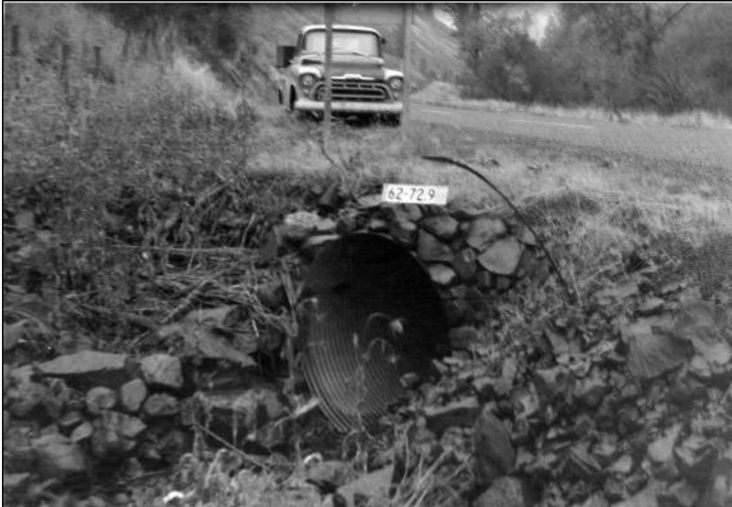
Figure 36. Culvert on ID-62 at Seven Mile Creek, built in 1938 by WPA. 241
