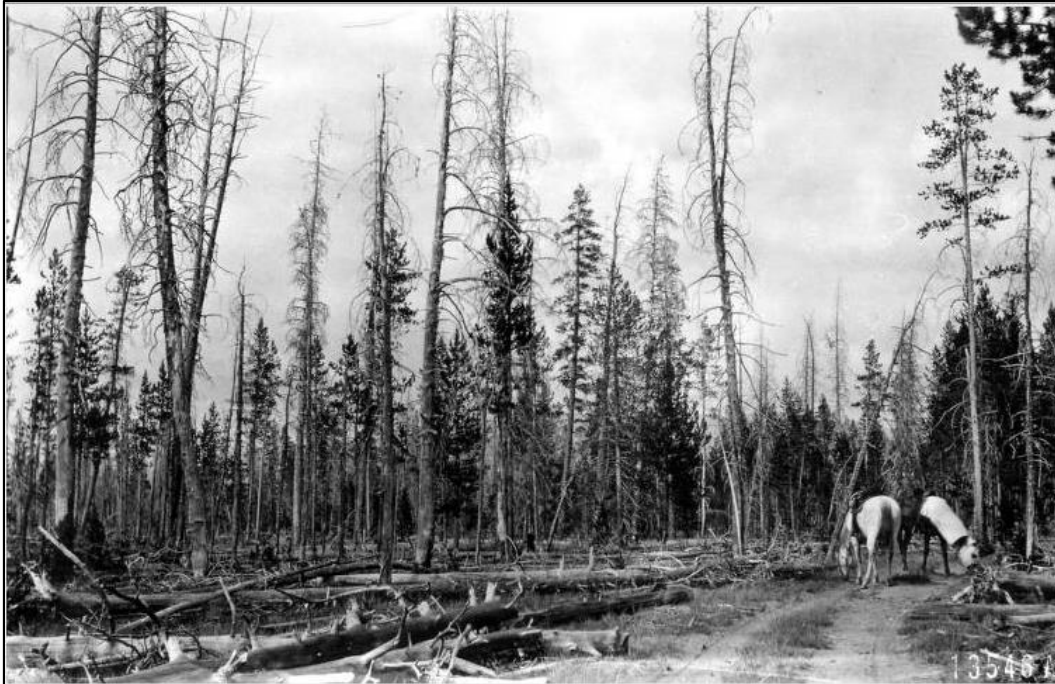
Figure 12. Bear Valley Wagon Road (north of Idaho City), c. 1912. 119
