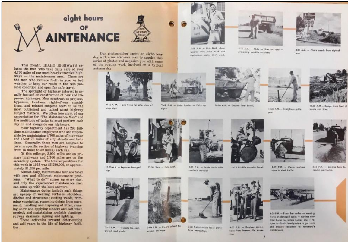
Figure 114. In the fall of 1959, Idaho Highway Magazine followed maintenance worker Orin Neth on a typical shift in which he picked up trash and debris, placed and replaced signs, and patched a segment of road. Neth was one of 280 full-time maintenance workers the highway department employed that year. 567
