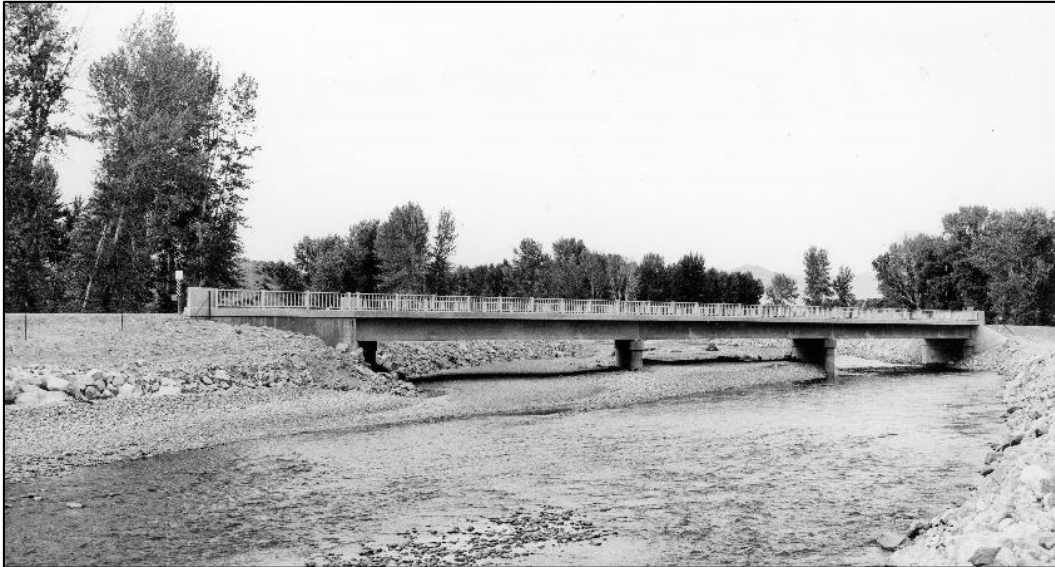
Figure 79. The Big Wood River Bridge, pictured in 1957, was the first use of prestressed-concrete girders in Idaho.
