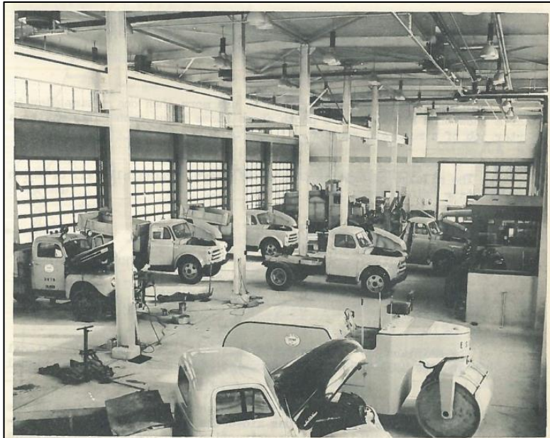
Interior of new District 6 Shop. Note ten ton overhead crane in far corner
