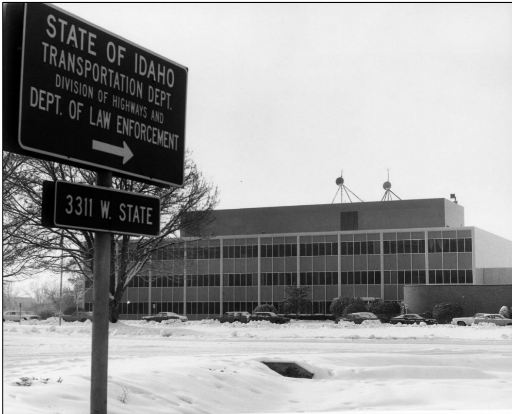
Figure 102. The new highway department building, begun in 1959 and completed in 1961, heralded a new era of communication and coordination. 518
