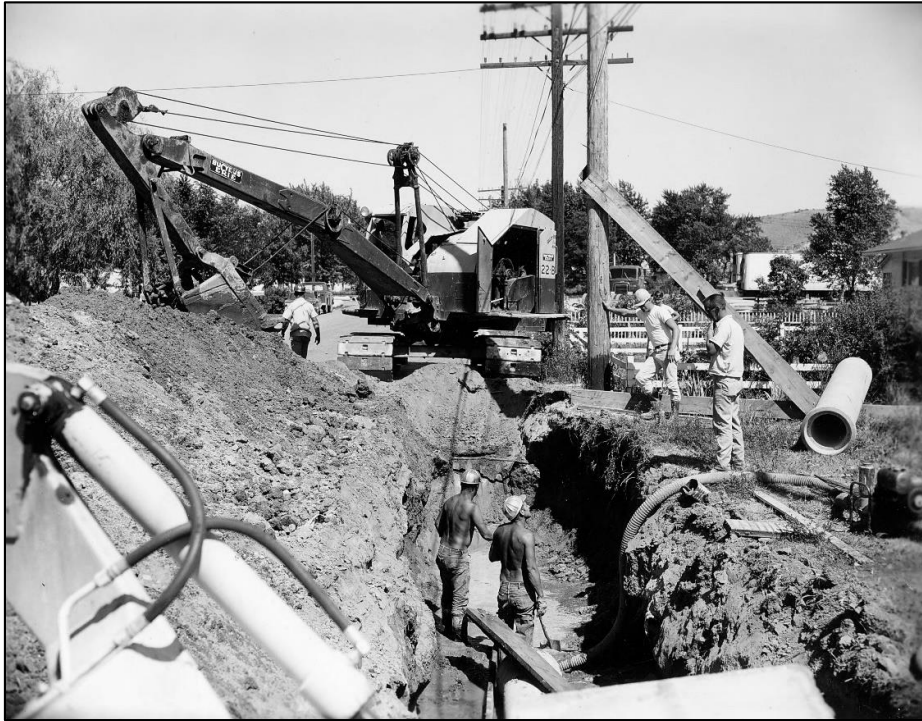
Figure 110. Road construction in Payette in 1966. 553
