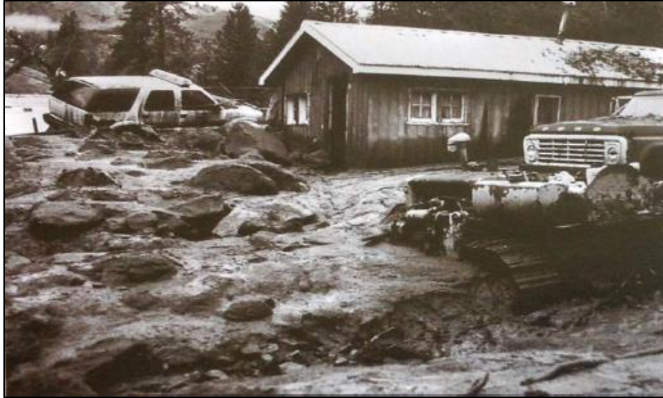
Figure 136. Historic flooding took place across the state in 1996 and 1997. The banks of the Payette River along ID-55 were one of the areas affected. 687
