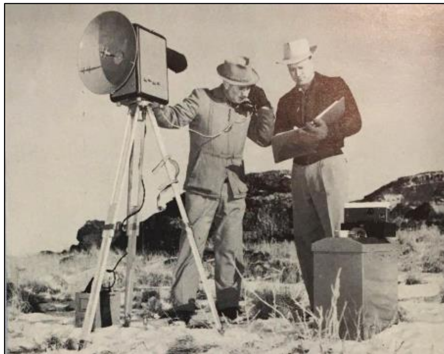
Figure 99. New technology helped the highway department meet increasing survey needs. The tellurometer, shown here, measured distances electronically and saved the highway department months of survey time. 508
