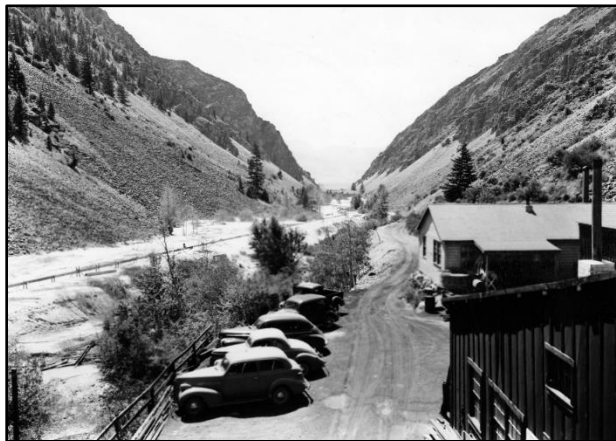
Figure 50. Access road to the Ima Mine in Lemhi County, c. 1940. 291
