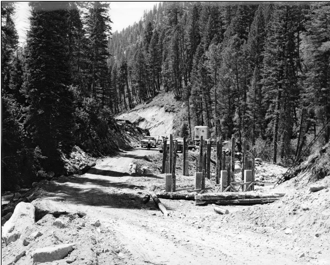
Figure 80. Forest Highway construction along ID-21 between Stanley and Lowman. 448
