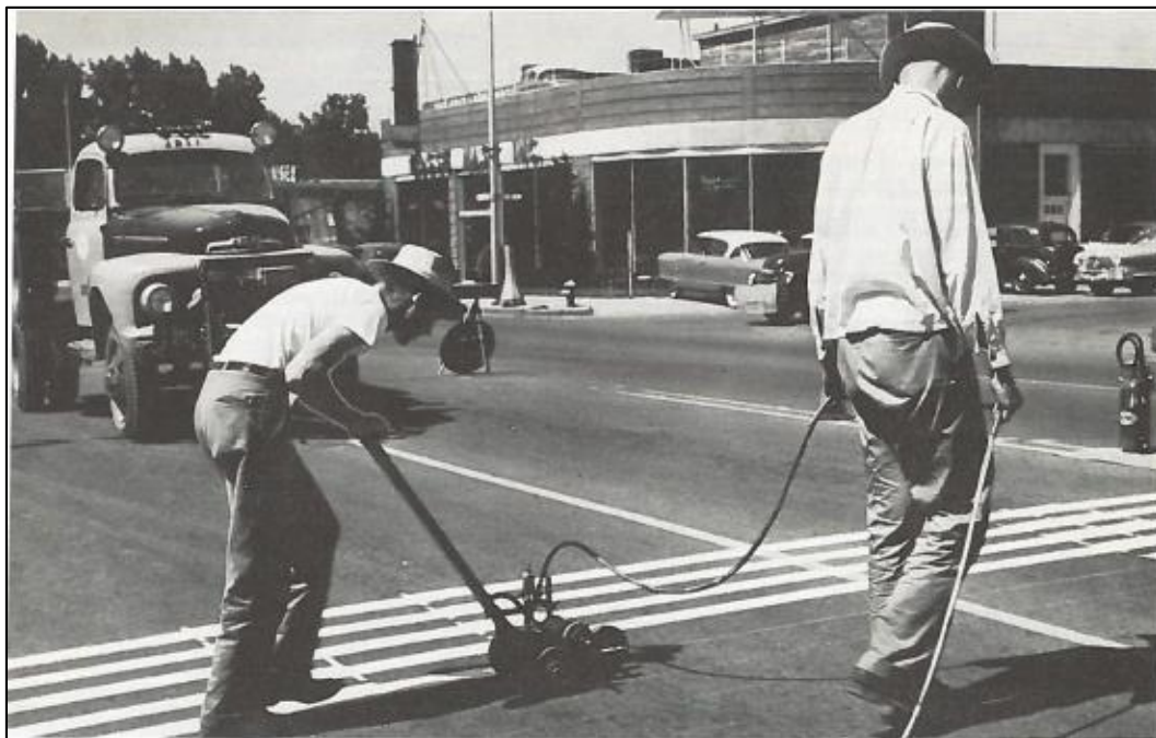
Figure 118. Department workers placing striping paint to test its durability in the late 1950s. 586
