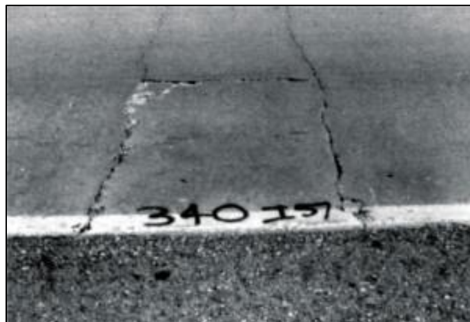
Figure 5 Edge Punch-out in CRCP
