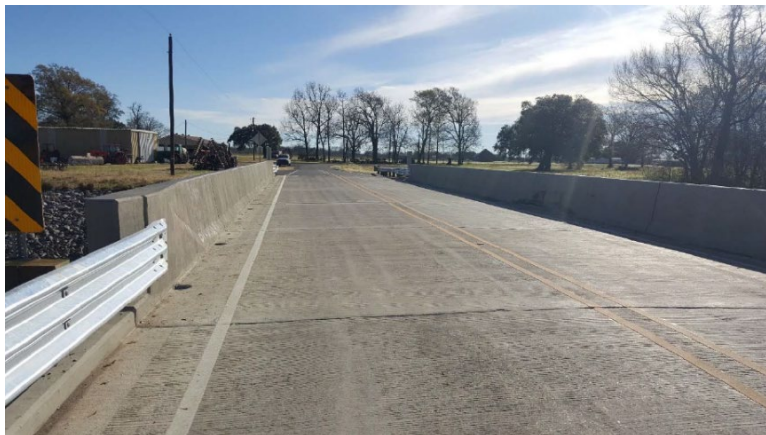
Figure 20. Internally cure concrete project at West Congress Street bridge
