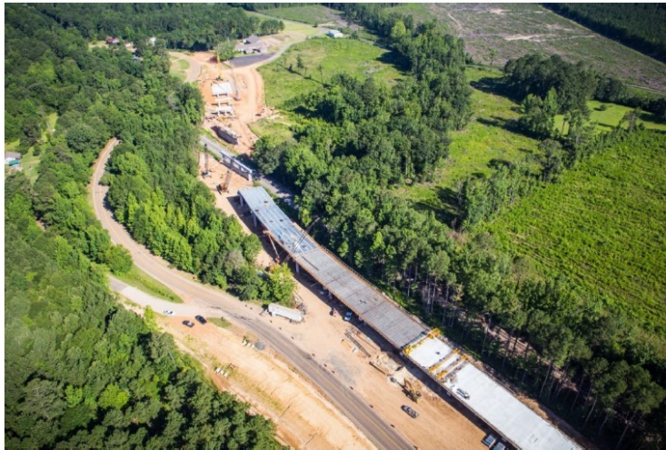
Figure 19. Internally cure concrete project at U.S. 80 near Ada, North Louisiana
