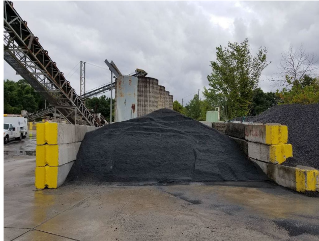
Figure 21. Stockpile of prewetted LWFA the day before placement of the internally cured bridge deck
