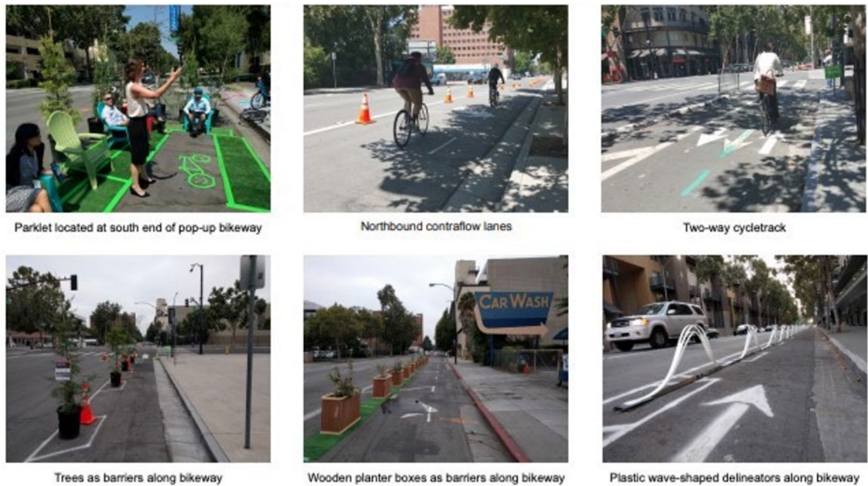
Figure 5. Different Complete Street Treatments in Downtown San Jose 49
