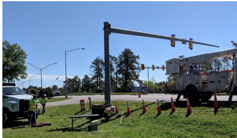
Figure 6. Pluck test performed on the overhead traffic signal
