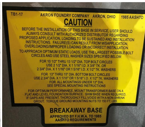
Figure 21. Electrical wiring (left) and manufacturer’s instructions for installation (right) inside T-base
