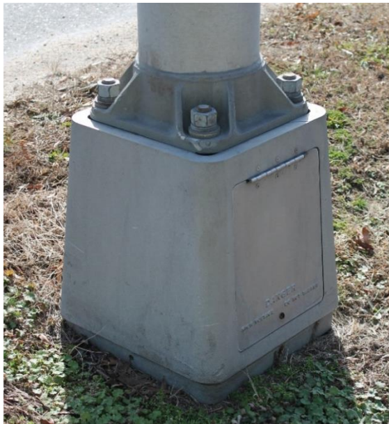
Figure 20. A luminaire with a T-base connection (left) and components including anchor rods (or bolts) inside a T-base (right)
