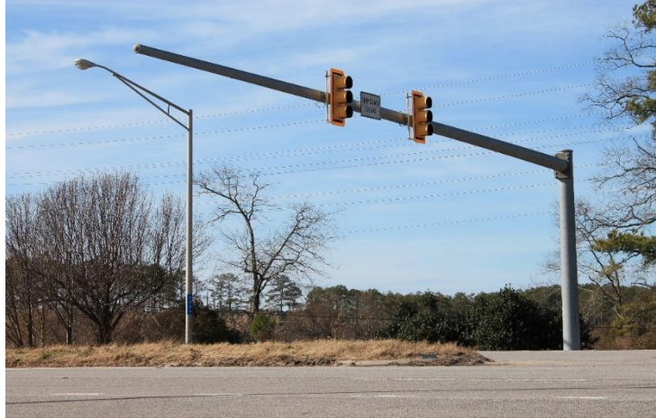
Figure 5. Instrumented luminaire and traffic signal near the east coast of Virginia
