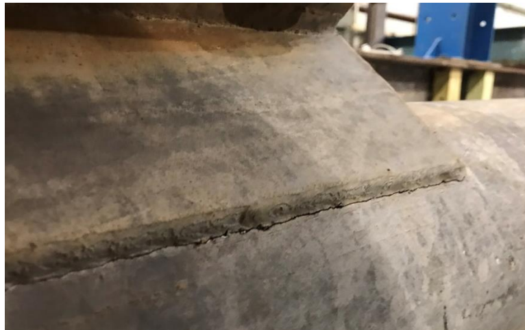
Figure 12. Fatigue weld crack at the box connection on the straight pole
