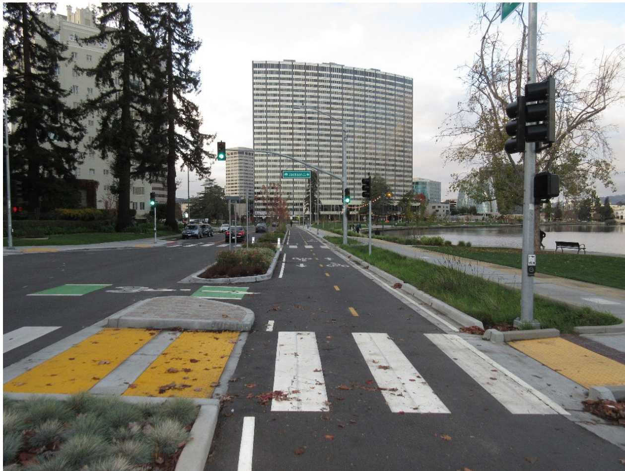
Figure 31. Looking North along Lakeside Drive in Oakland, the pedestrian path on the far right is separated from street traffic on the far left by biostrrips, street trees, and a class IV bikeway in the middle.
